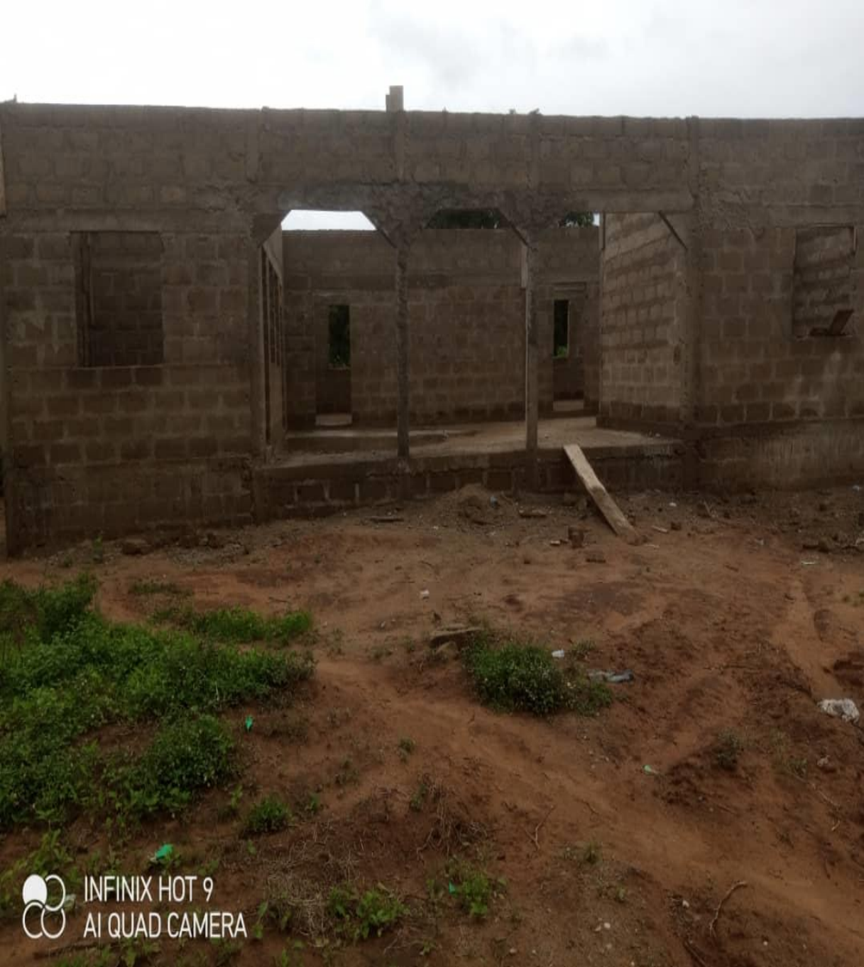
Constructed a 1 No: CHPS Compound -LENTIL LEVEL
