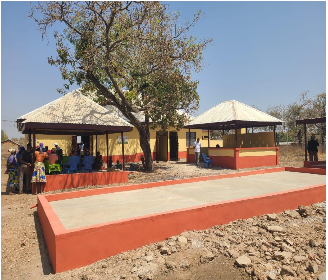
Rehabilitation of shea processing facility at cache
