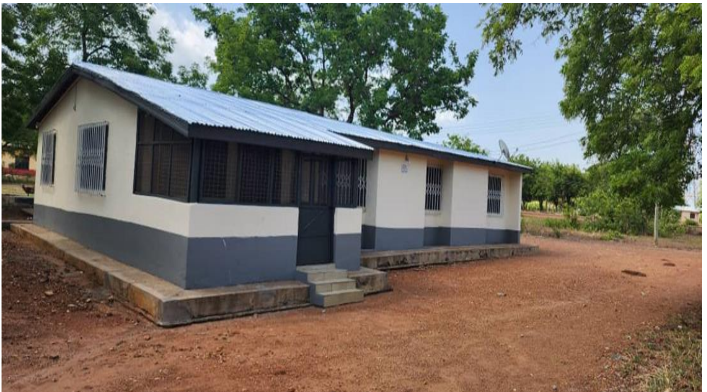
Renovated Bungalows for staff
