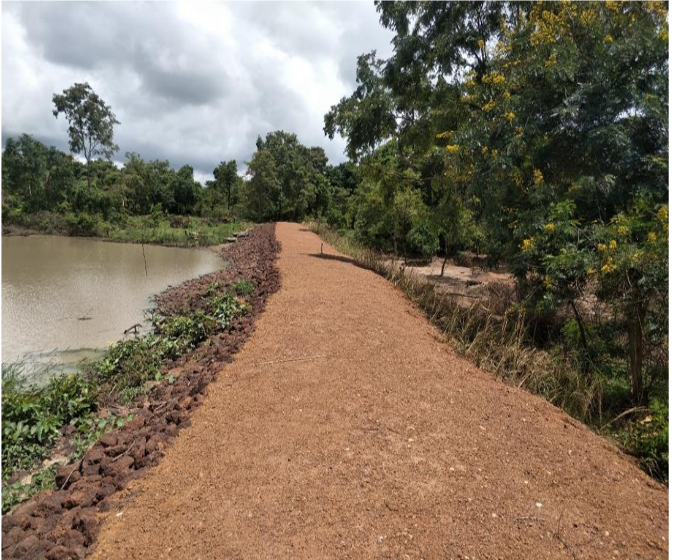
Rehabilitated Sonyor Small Earth Dam
