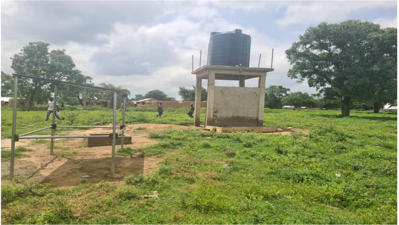
2NO. Solar powered mechanized boreholes constructed at Dikatama and Gbebiri
