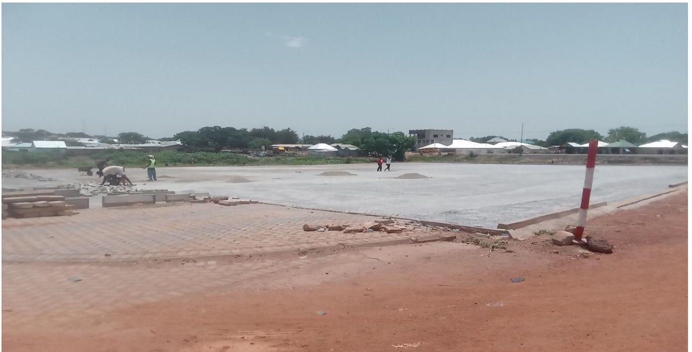
Constructed Lorry Park at Gbenfu Junction
