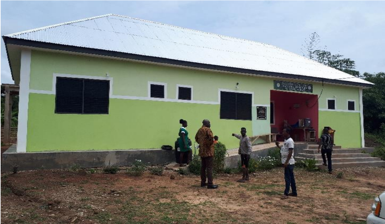
Completed 1no. CHPS Compound with 2-bedroom Nurses' Quarters at Akaa
