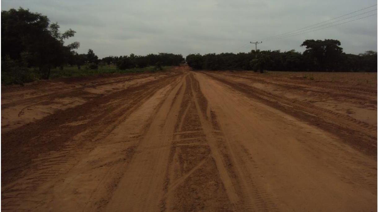
Reshaped Bunglung-Tumahi and other feeder road (5.00 km)
