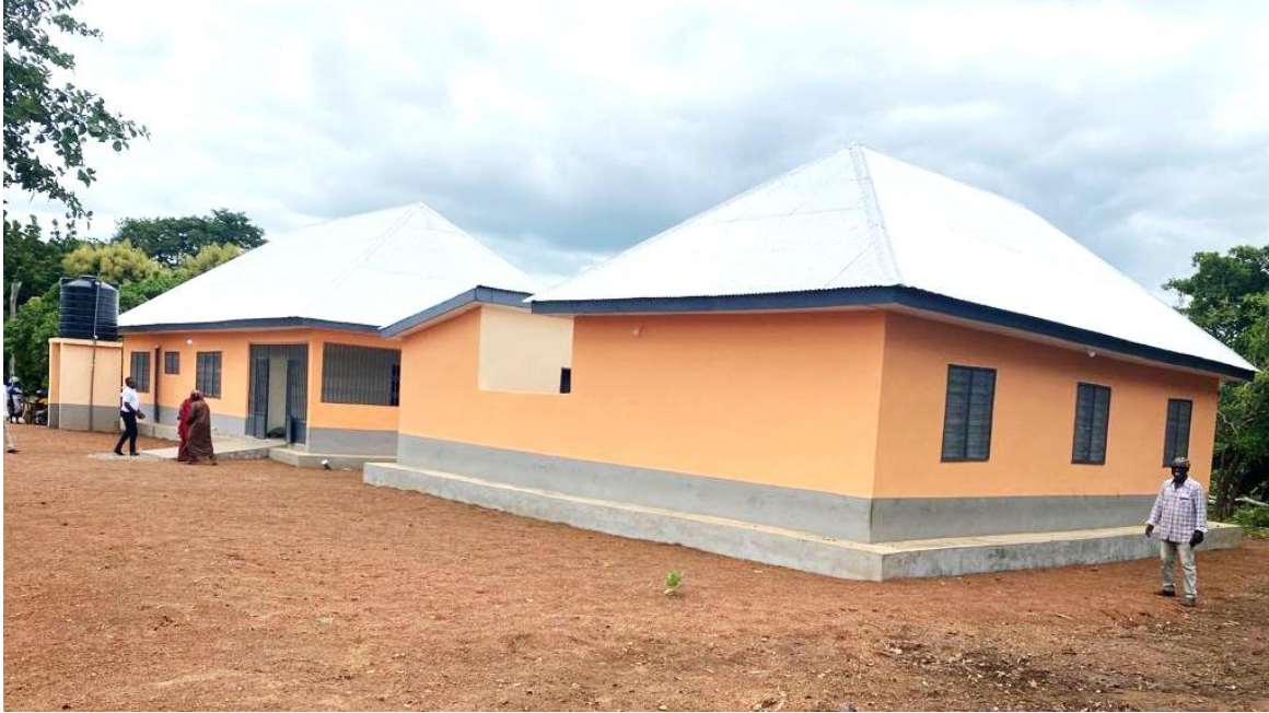
Figure 6: Constructed 1No. CHPS Compound with 3-Bedroom Accommodation and 1No. 2-Seater KVIP Toilet at Gambuga
