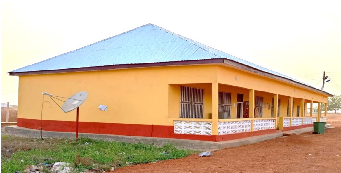
Figure 9: Rehabilitation Electoral Commission Office in Bimbilla
