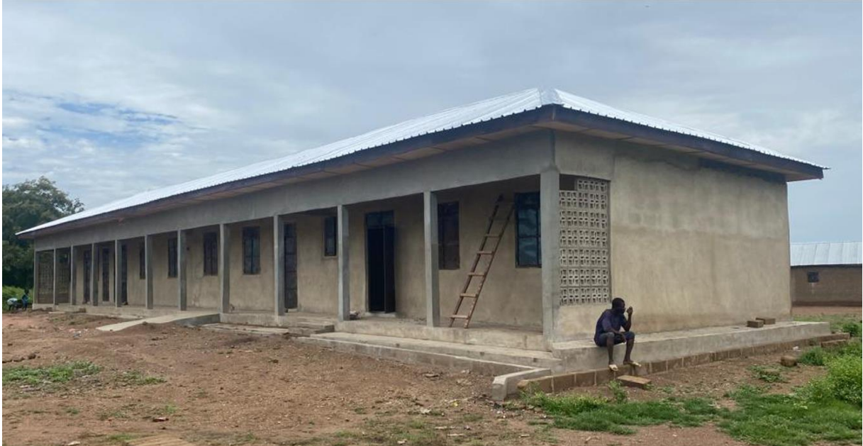
Figure 4: Constructed 1No. 3-Unit Classroom Block with Ancillary Facilities at Nchimbado
