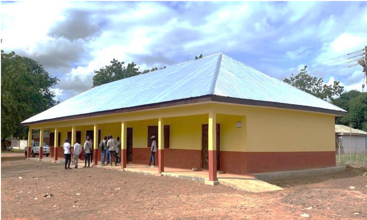
Figure 5: Rehabilitated and furnished 1 No. 3-Unit Classroom at Presby Primary School, Bimbilla
