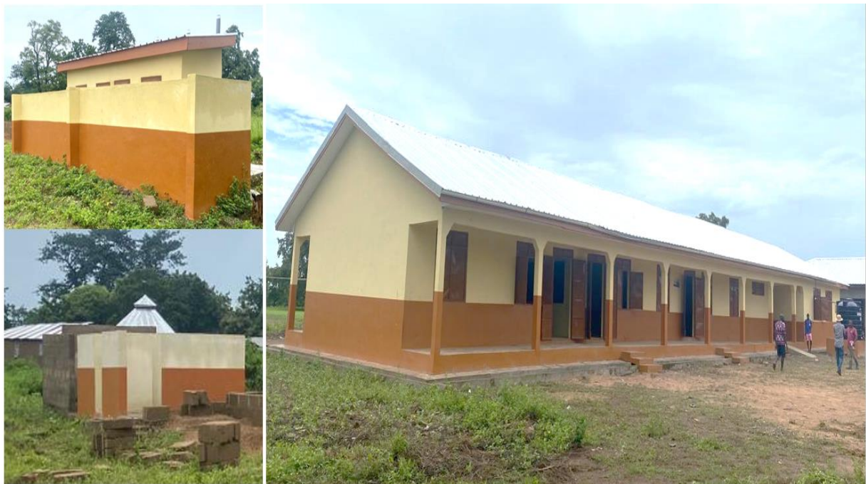
Figure 3: Rehabilitated and furnished 1 No. 3-Unit Classroom at Nchimbado
