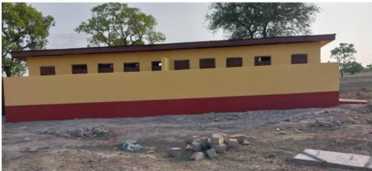
COMPLETED 8 NO. KVIP TOILET WITH 2NO. CHANGING ROOM AT GAA MARKET
