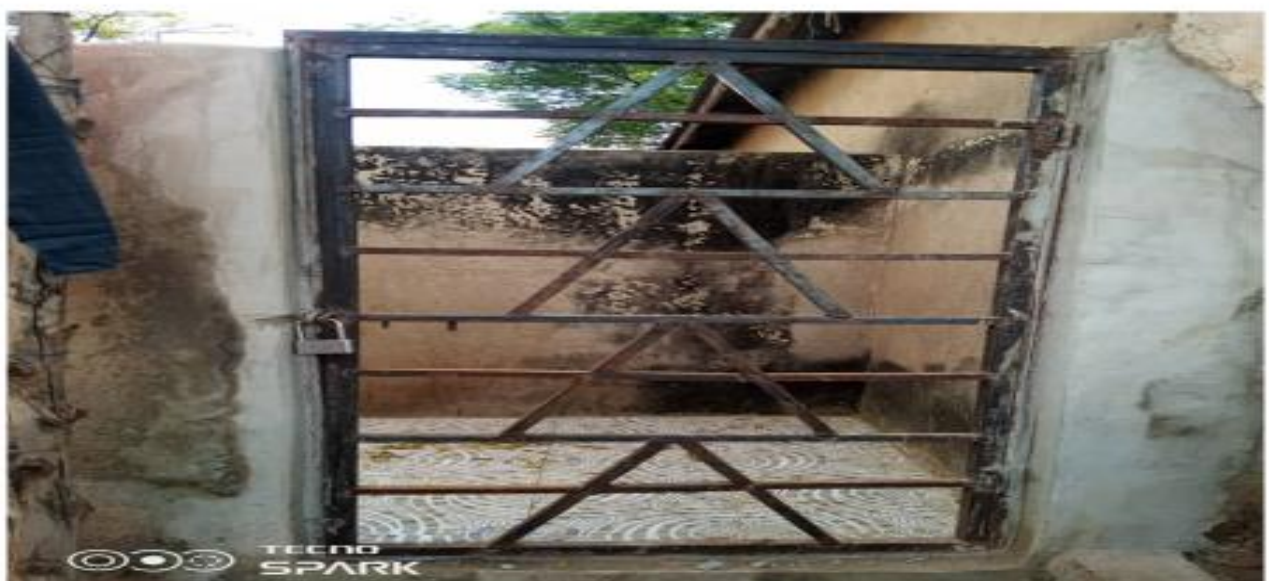
Rehabilitation of 2 unit urinal at Gushegu market-on going under IGF
