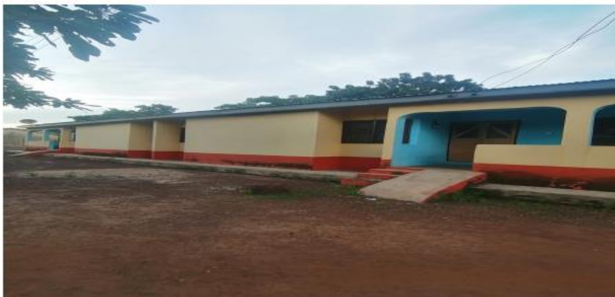
REHABILITATED STAFF BUNGALOW AT GUSHEGU
