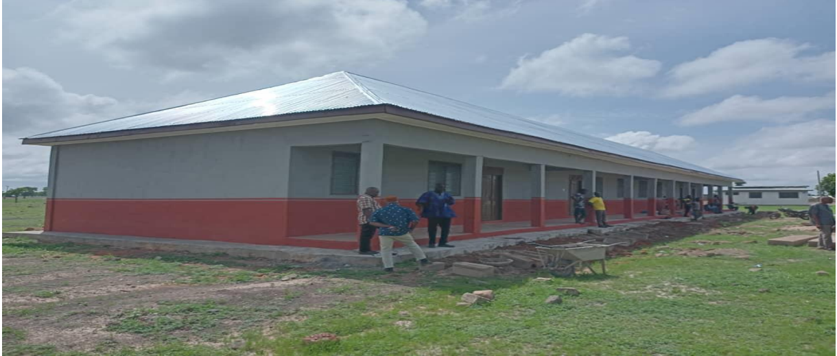
Constructed and furnished 1No. 3-Unit Classroom Block at Gbintiri SHS
