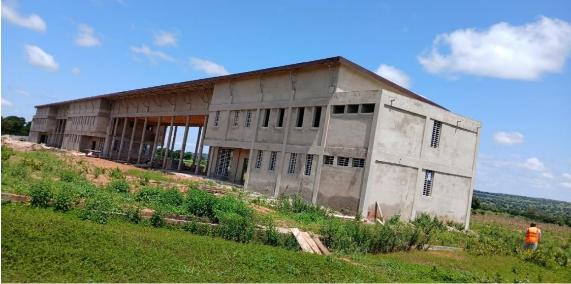
• Complete Construction of Bus Terminal, Public Washrooms and Paving at Nalerigu
