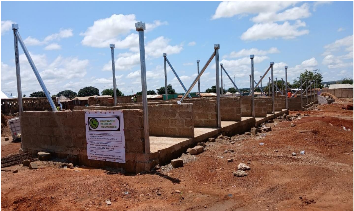
Construct 20-seater Toilet, 30no. Stalls and External Works, at Nalerigu
