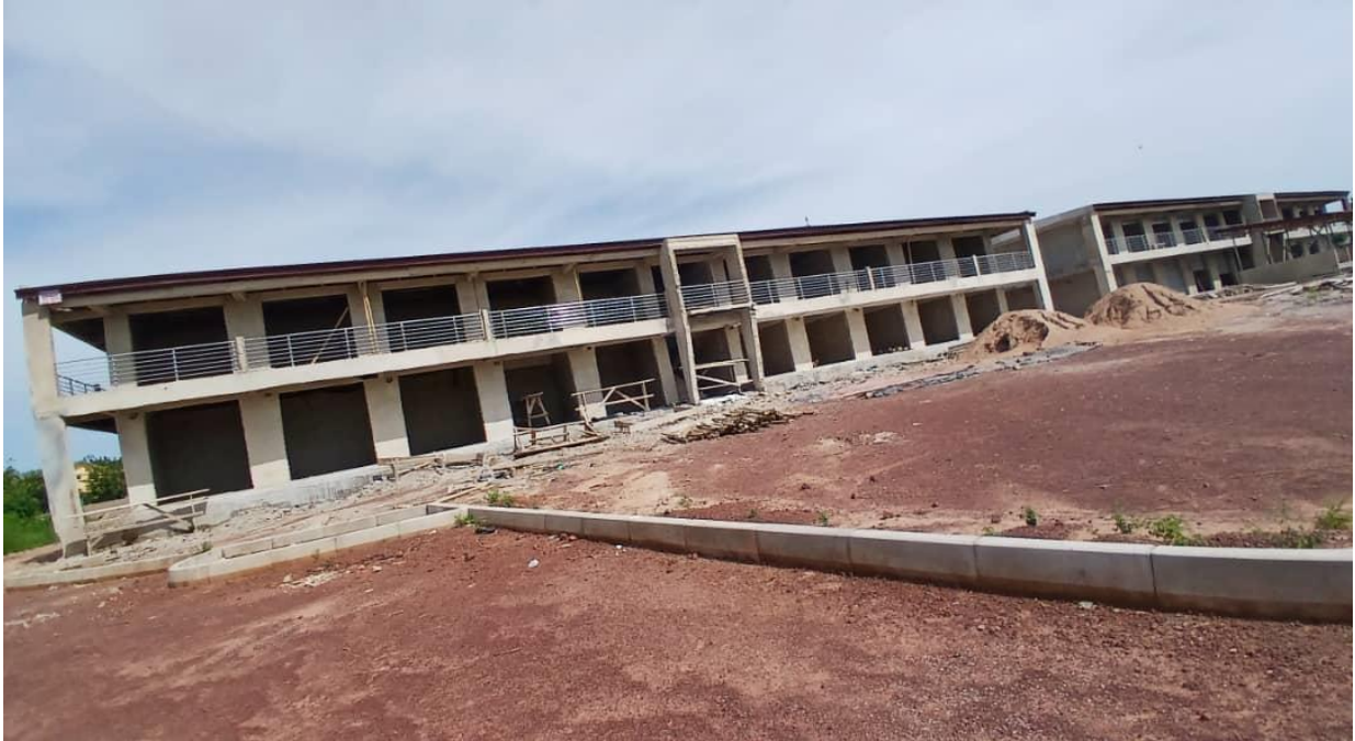
Construct two-storey 80 lockable stores at Gambaga
