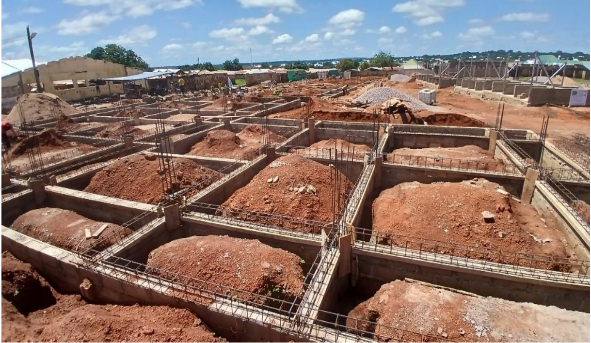
Construct two-storey 80 lockable stores at Nalerigu
