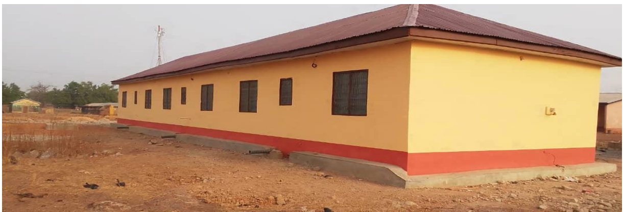
Constructed and furnished 1No. Teachers Quarters at Tuni
