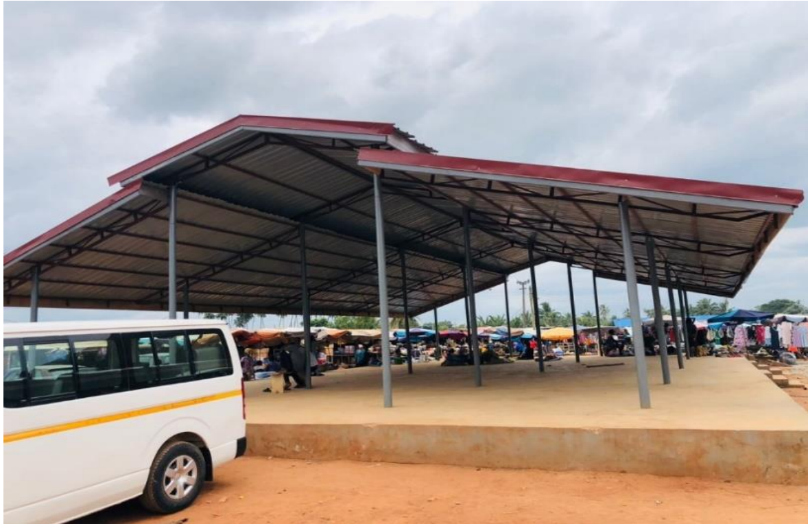
Completed 2No. 36 open shed at Dodowa Market
