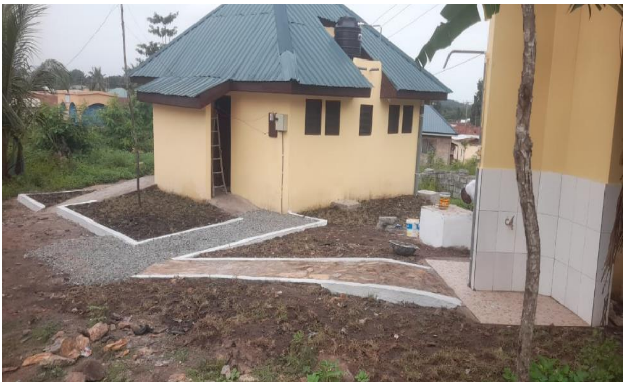
Completed 10-seater WC with Mechanised borehole at Agomeda
