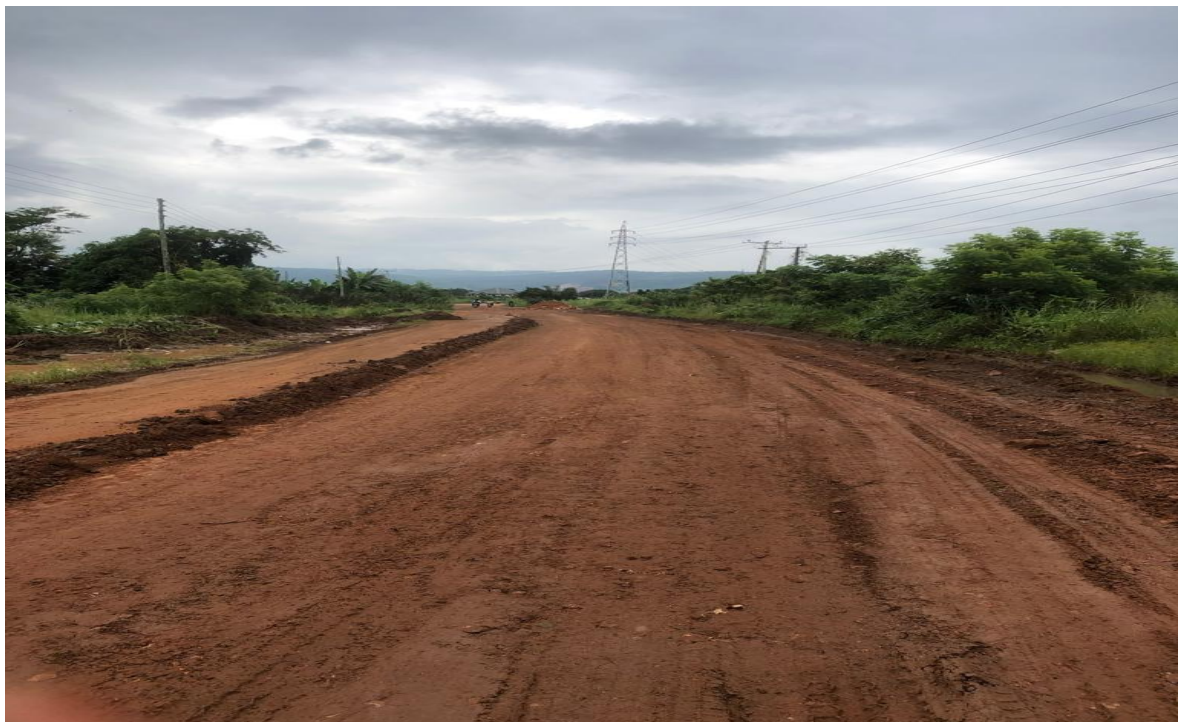
Reshaped and Graveled Ashiaman Junction-SOTA Road.
