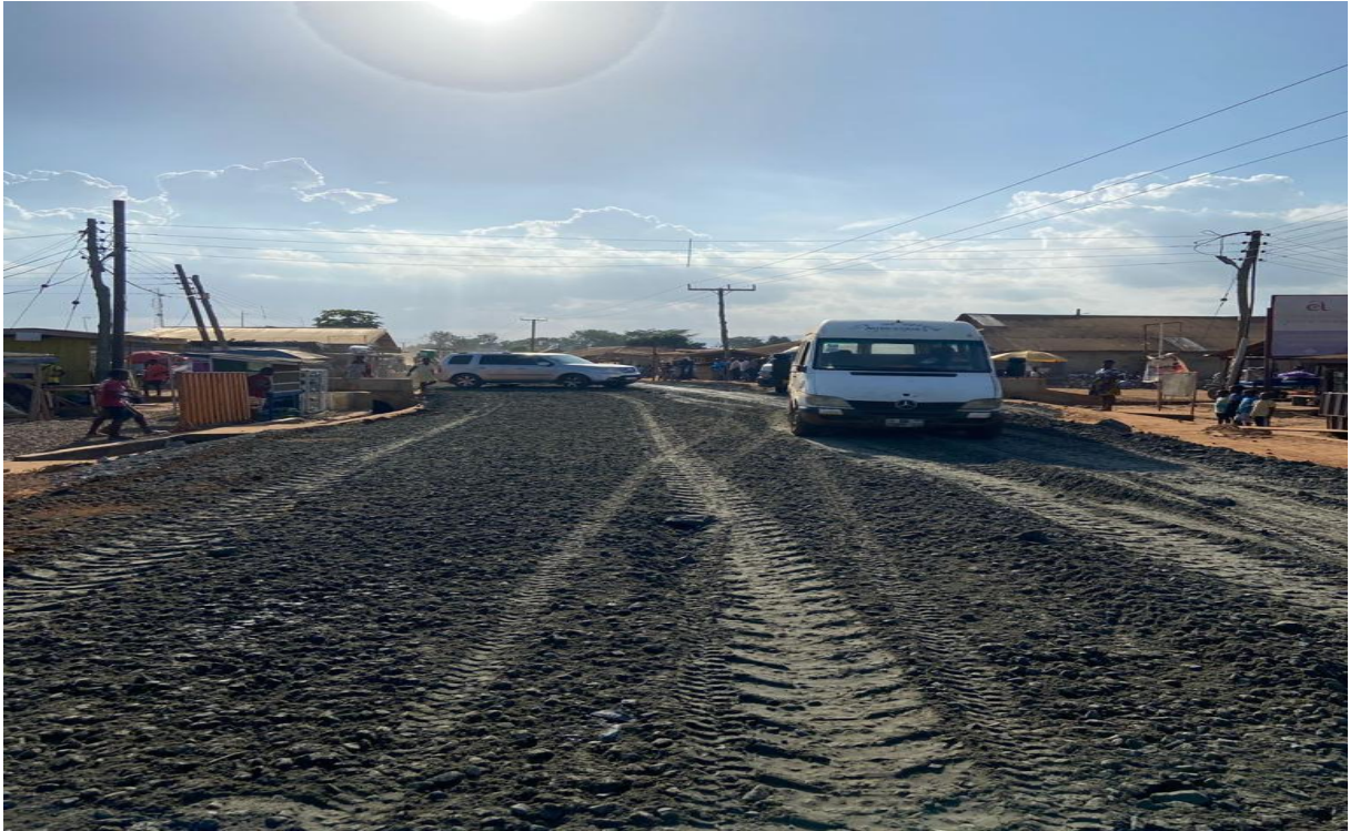
Reshaped and Graveled Doryumu-Shai hills junction road
