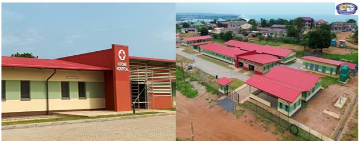
Constructed 40 bed capacity Hospital in Kpone
