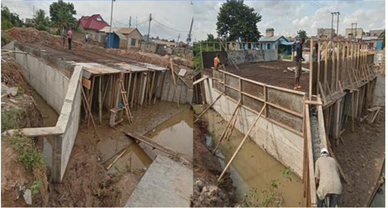
Constructed of 2 x 3.5M box 3 cell culvert at Prime Bar, Kubekro
