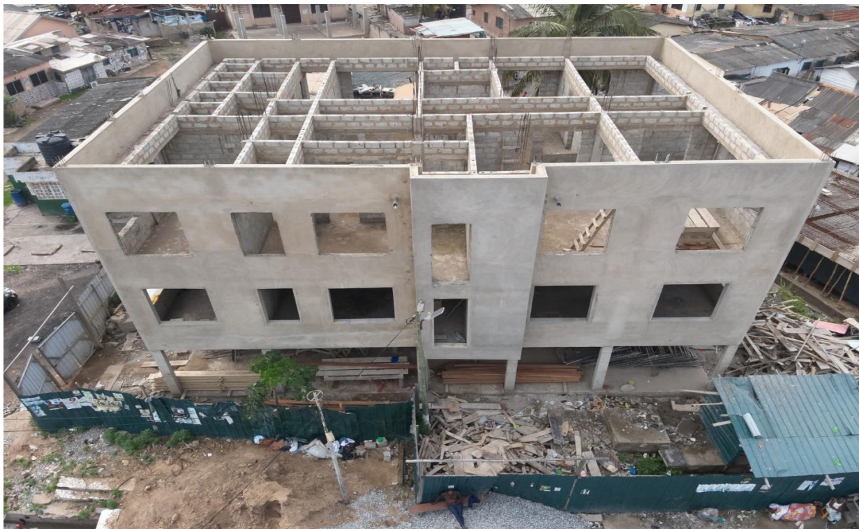
CONSTRUCTION OF ZONAL COUNCIL OFFICE COMPLEX AT OSU
