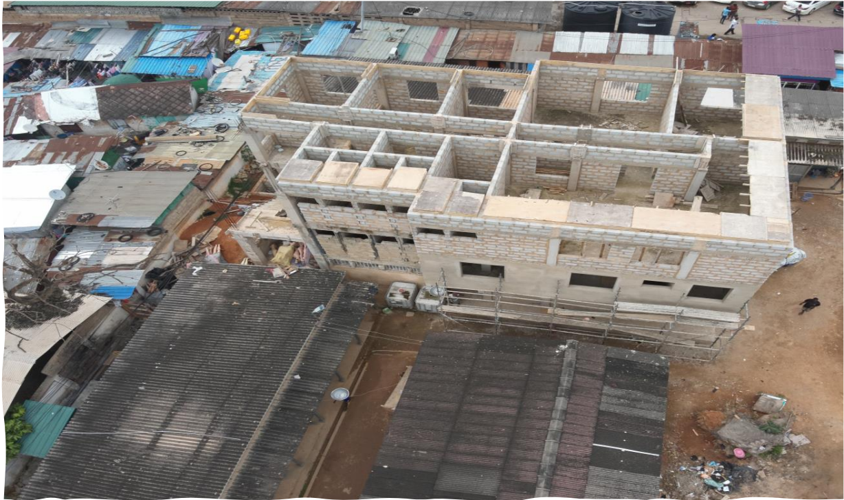
Construction of 3 Storey Zonal Council Office at Adabraka
