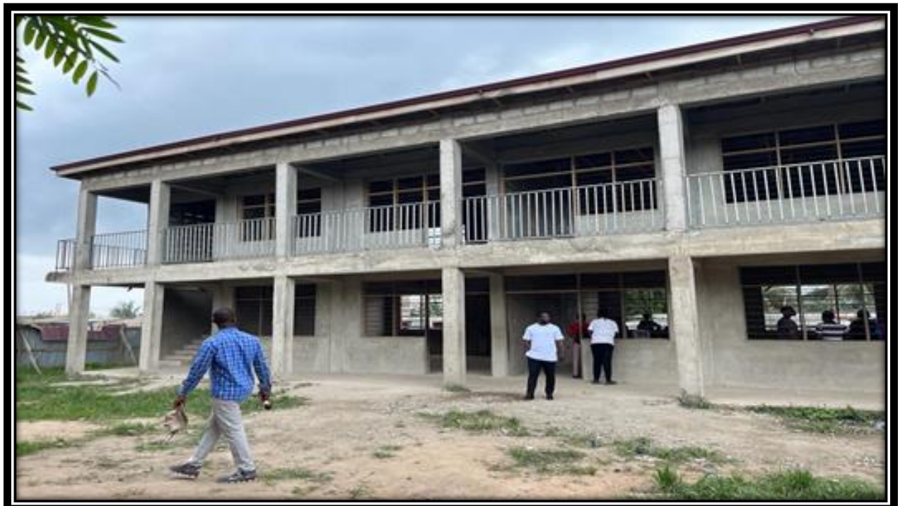
Construction of 2-Storey 6 Unit Classroom Block at Ashalaja
