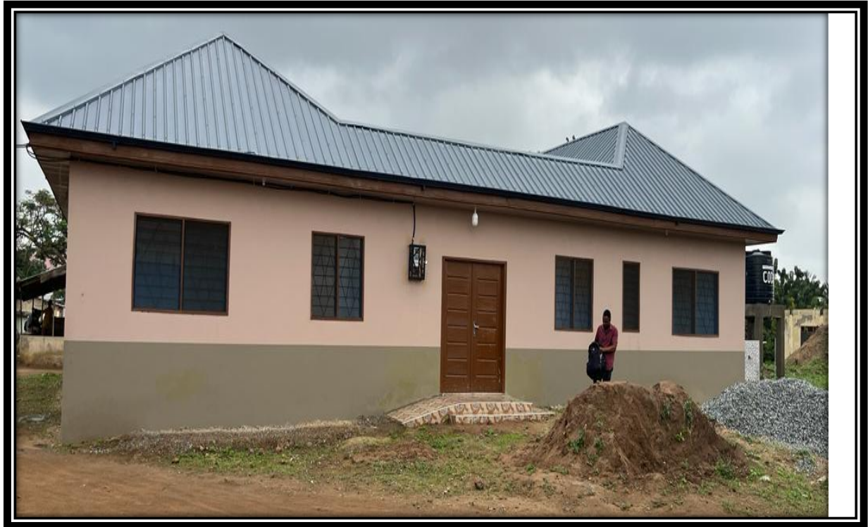
Completed CHPS Compound at Domeabra
