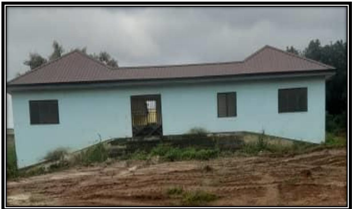
Completed CHPS Compound at Fankyenenko
