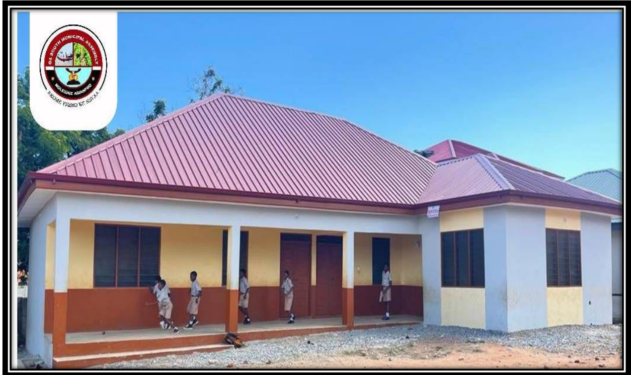
Completed 1 No.2 Unit KG Block at Bortianor
