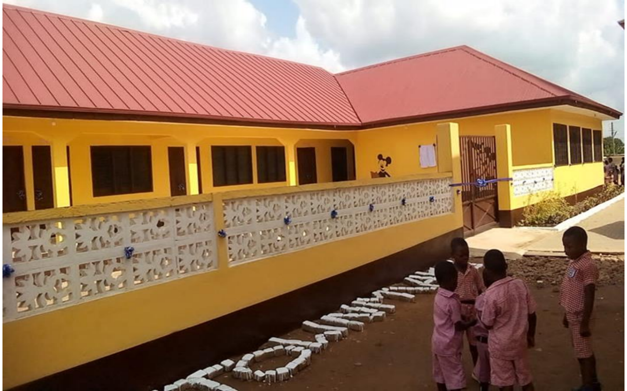
Construction and furnishing of 1no. 3-unit kg and nursery classroom block at Newtown- Suhum
