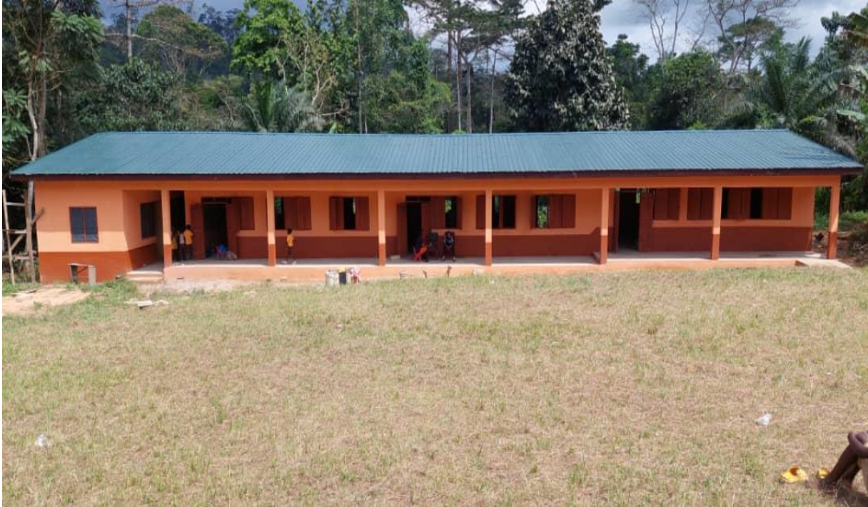
Constructed 1no 3unit Classroom block with ancillary facilities at Gyaekasa
