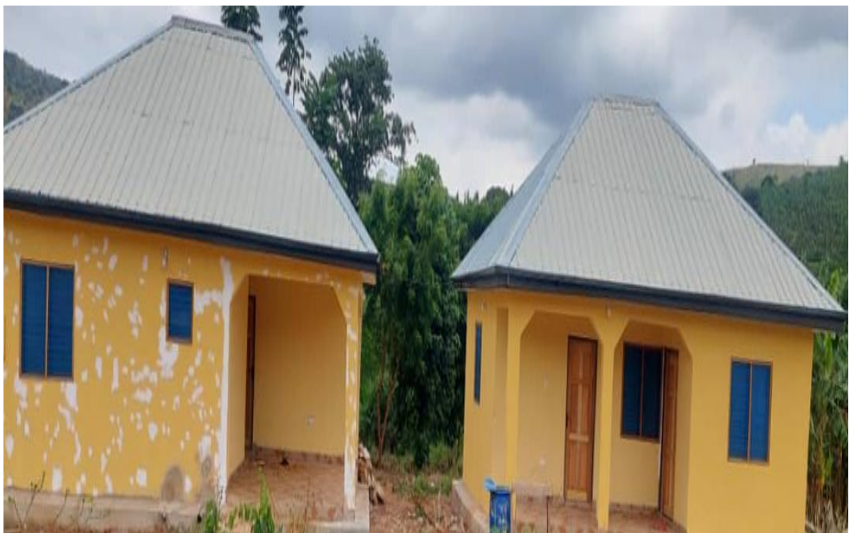
Figure 3 Completed 1No. 3-Unit Classroom Block, Urinal, KVIP and Office at Kwahu Tafo.
