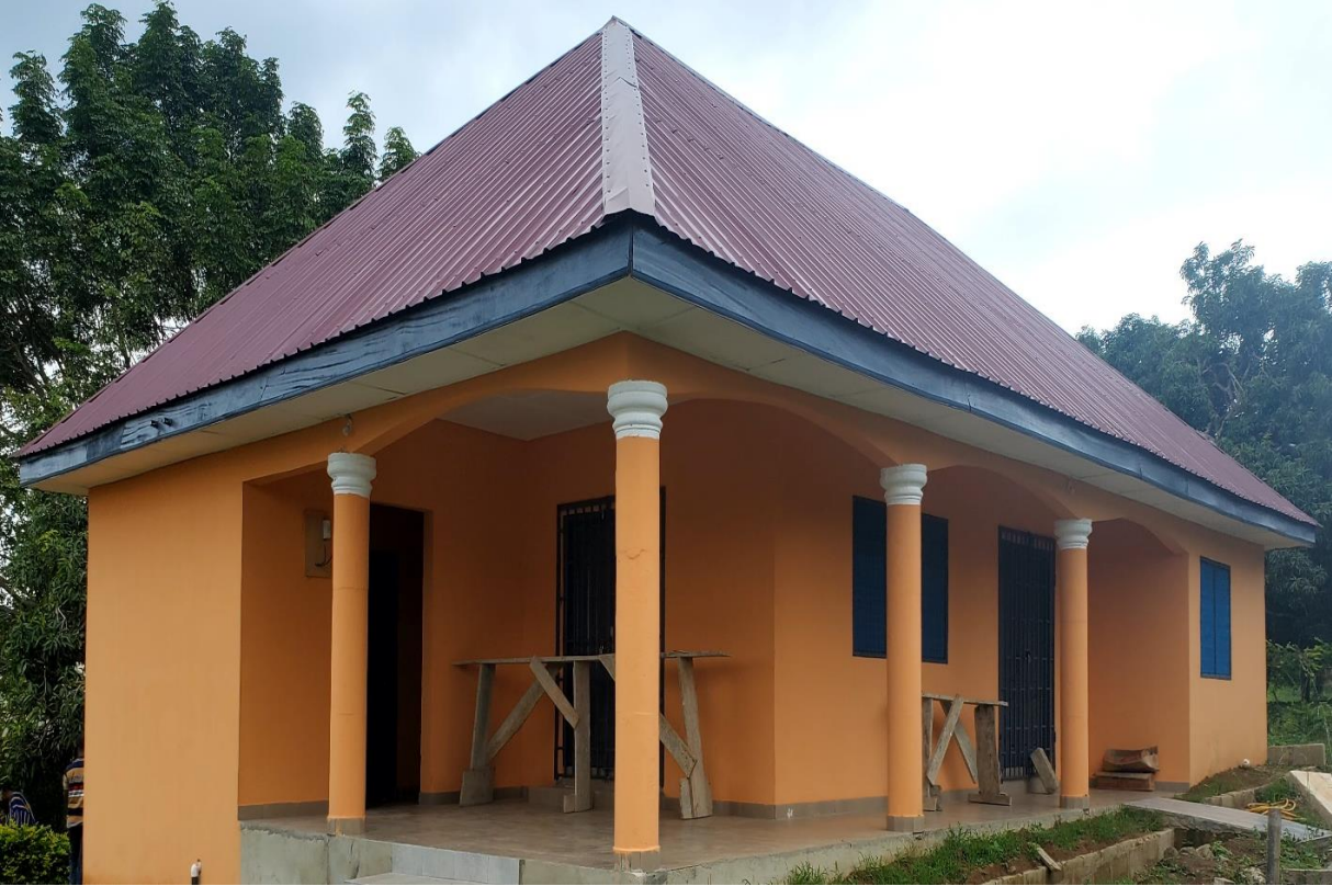
Figure 9 Completed 2No. 24-Units Market Shed at Pepease
