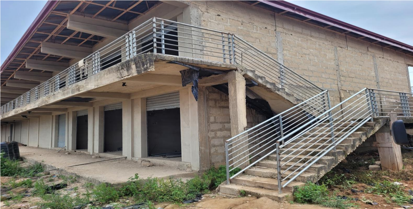
64 LOCKABLES STORES @ NEW ABIREM (80% COMPLETION)- IGF FUNDED
