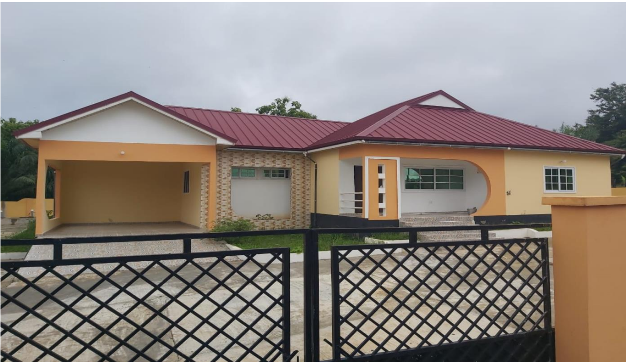
RENOVATED DISTRICT MAGISTRATE RESIDENCE AT NEW ABIREM
