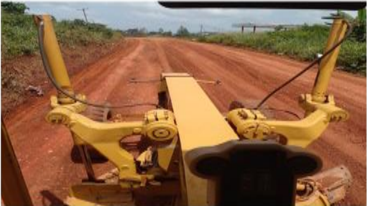
Reshaping of 55km feeder roads
