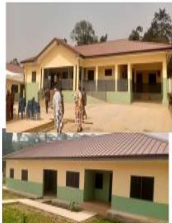
Health Facility with Accommodation at Nkroful 27
