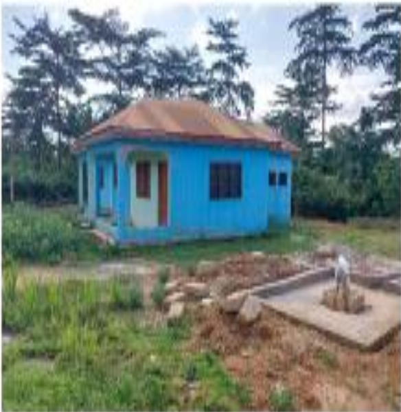
Construction of CHPS Compound at Aburi With mechanized borehole
