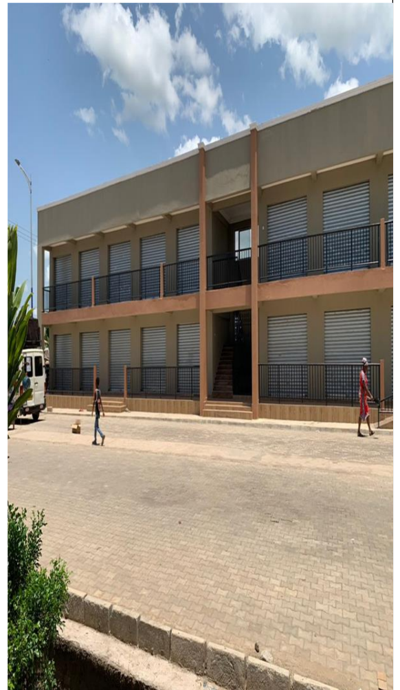
20 Lockable Stores at the Ansa Park, Mankessim (UDG 3)
