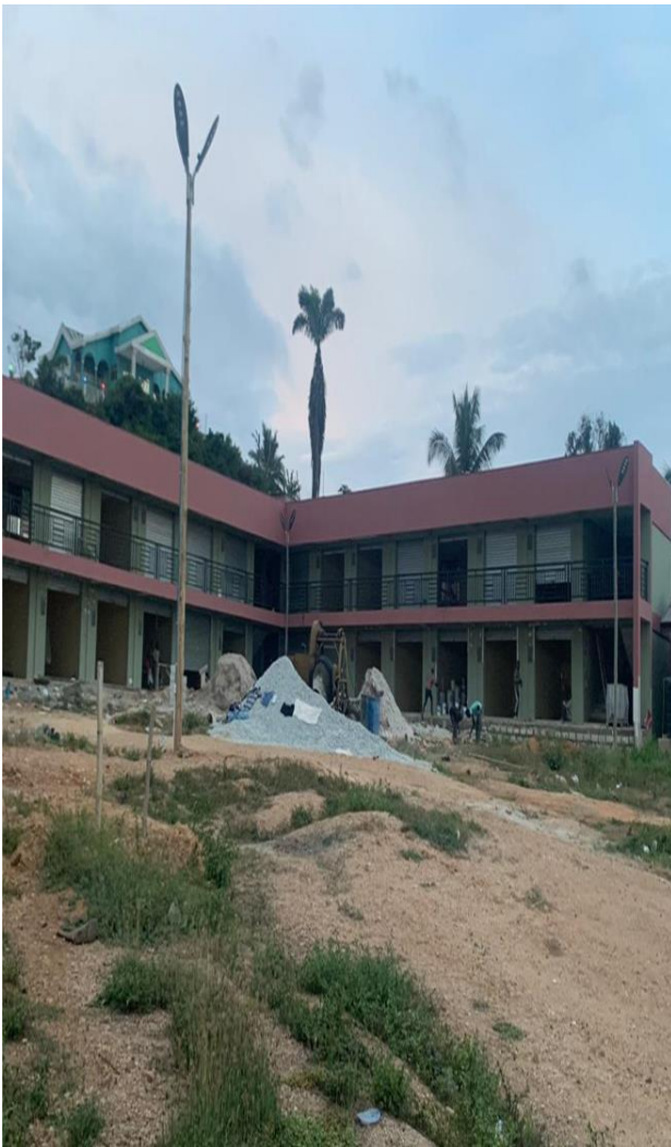
Construction of 60 No. lockable stores at Anomabo
