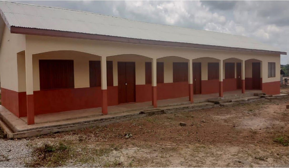
Figure 2: Construction of 1no. 3unit classroom block at Appiakrom Debiso
