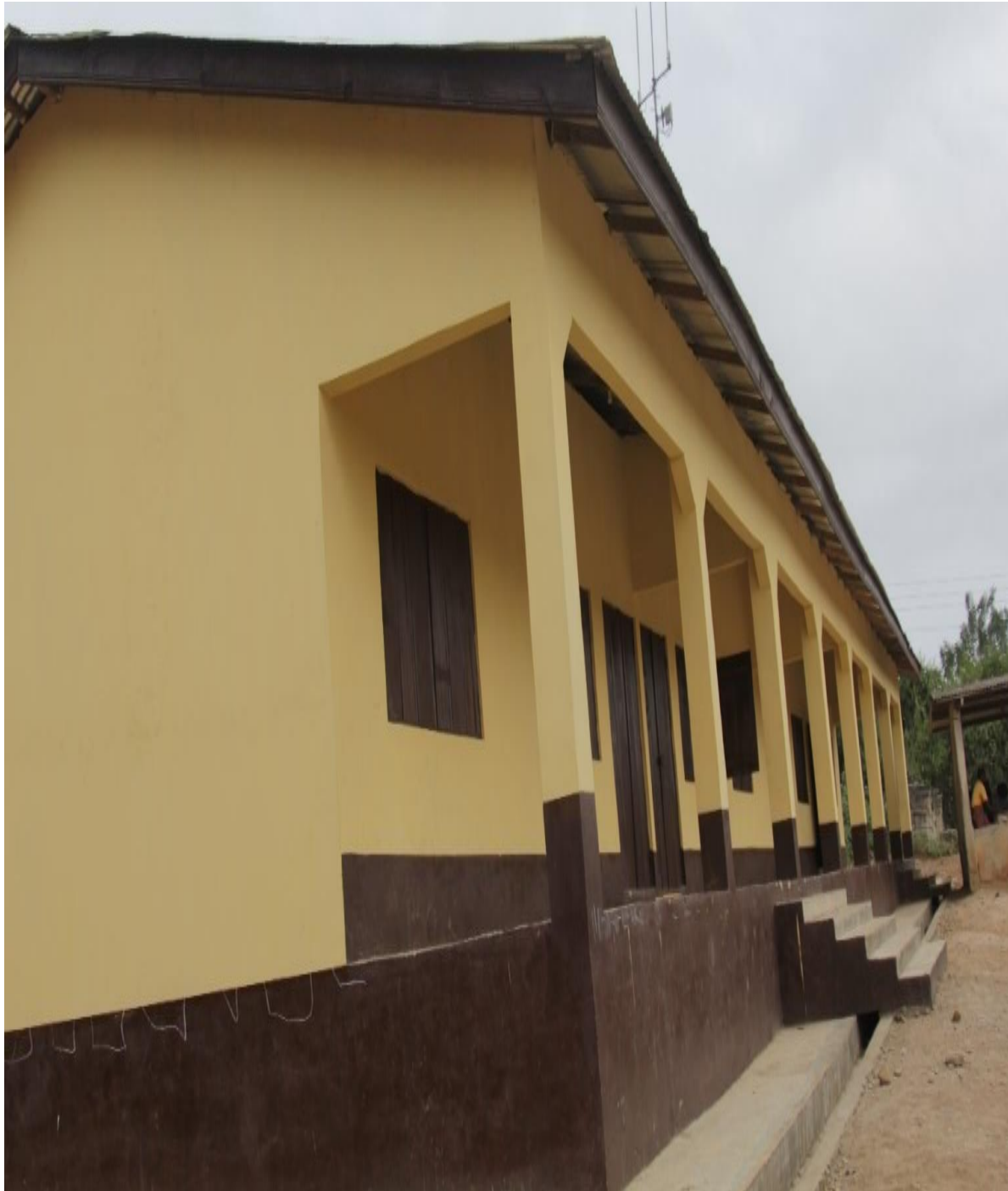
Figure 1: Construction of 1No. 3 Unit classroom block at Gomoa Obiri
