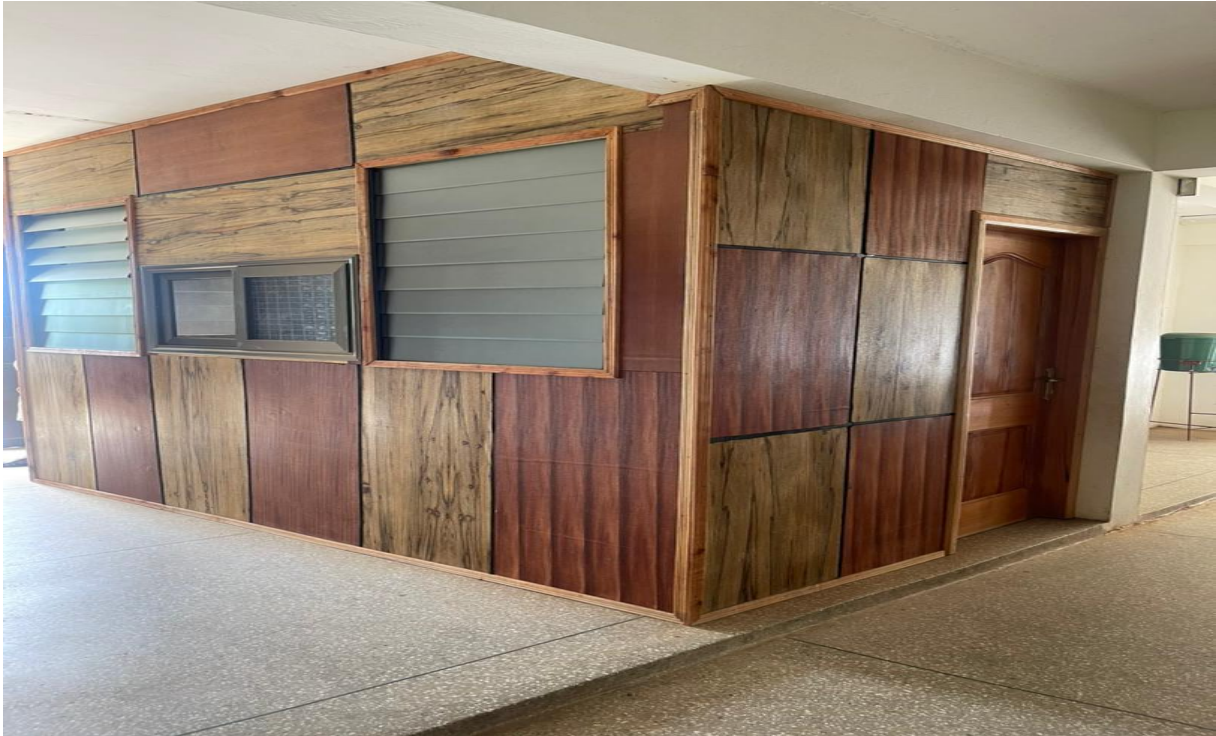
Figure 4: Construction of client service office at the district assembly
