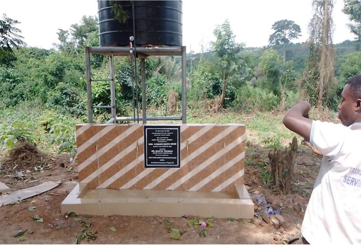
Figure 3: Construction of 7No Mechanized Boreholes within the district
