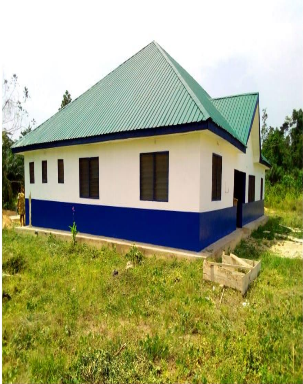
CONSTRUCTION OF 1- NO. POLICE STATION - ASSIN BEDIADUA
