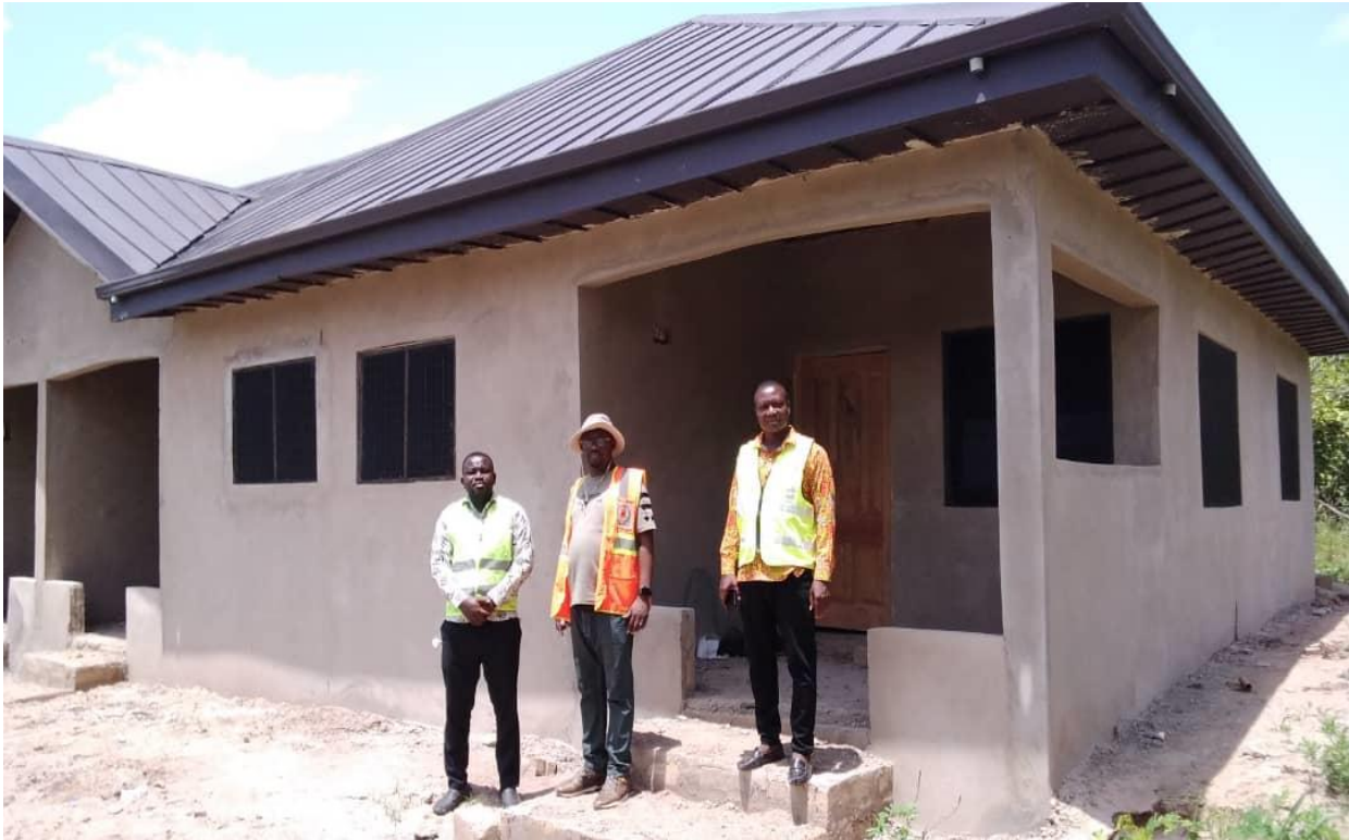
Figure 2: Constructed Police post With Staff Quarters at Nchiraa
