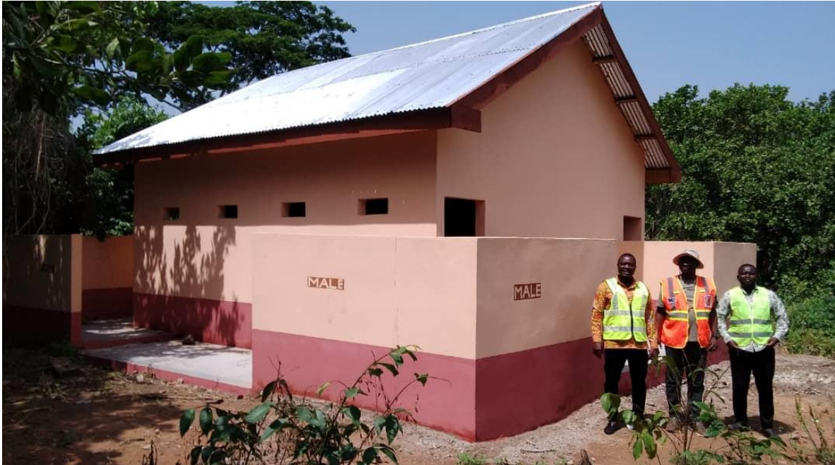
Figure 1: Constructed 6-Unit Aqua Privy Toilet at Akete (MP Fund)
