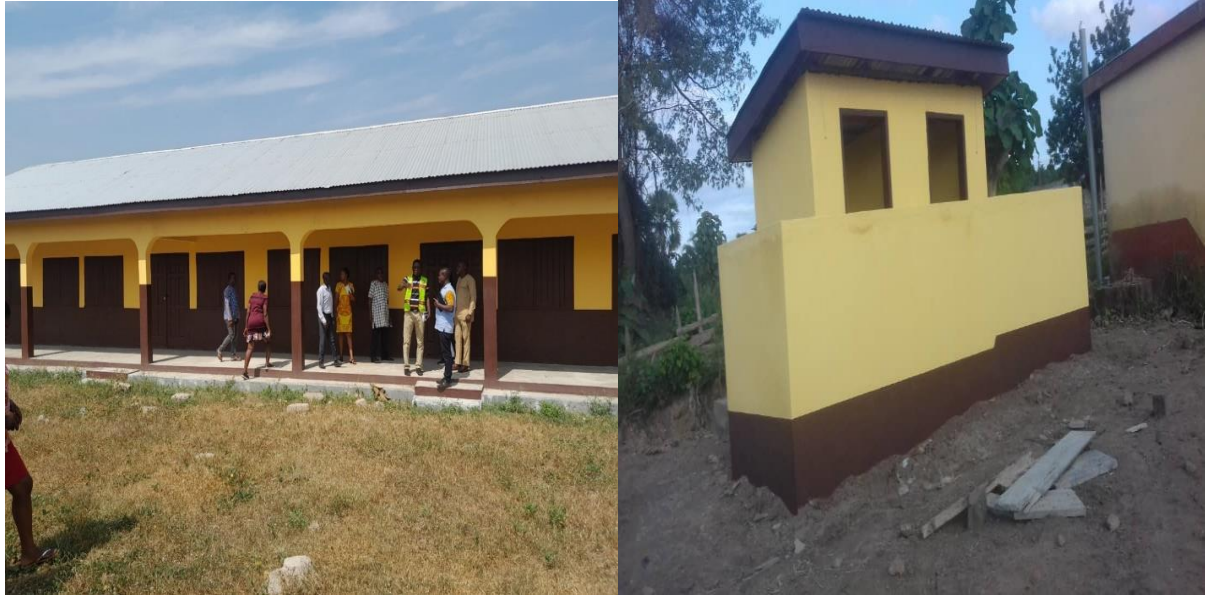
Figure 7: Constructed 1No. 3-Unit classroom block with ancillary facilities for M/A JHS at Twumkrom/Amoakrom.
