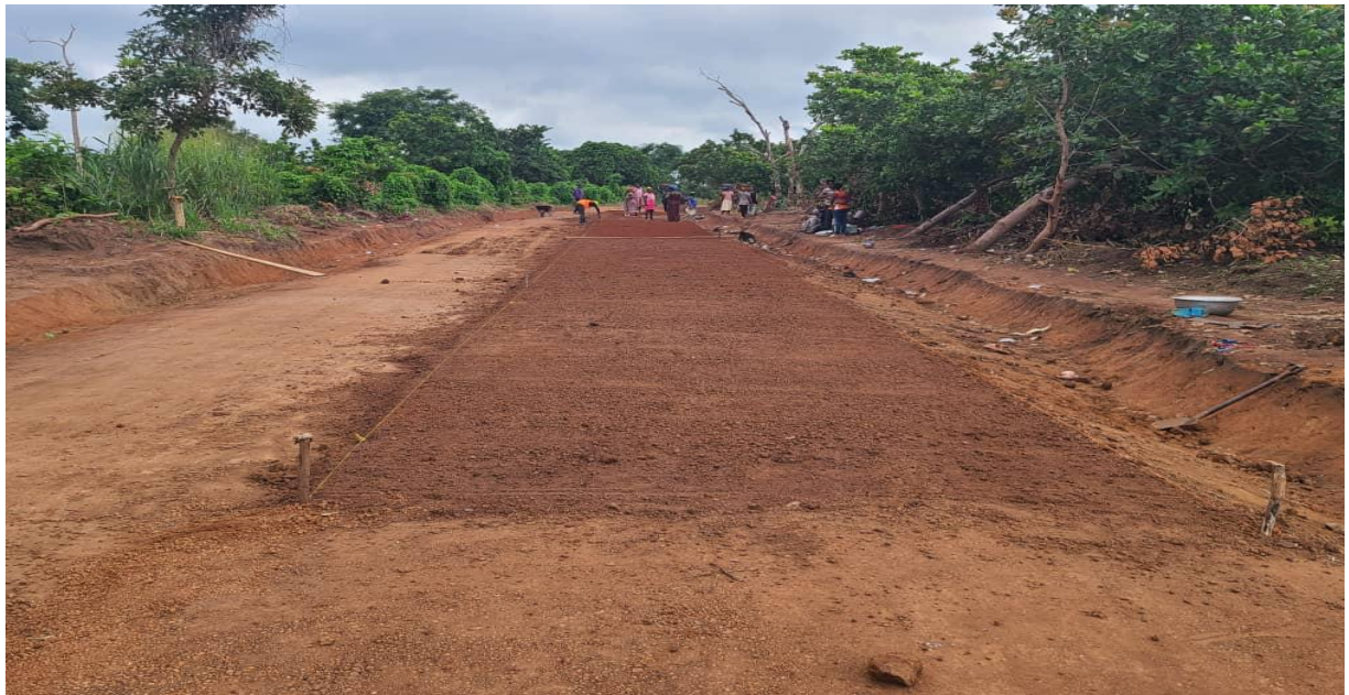
Figure 8: Constructed of 4.8km Nwoase-Seidu Akuraa-Congo-Aboabo Feeder roads using LIPW
