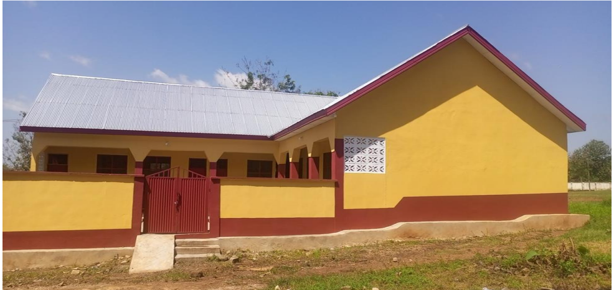
Constructed and furnished 1No. 2-Unit KG Classroom Block with Office, Stores, Ceiling, Wiring at Stadium Basic School
