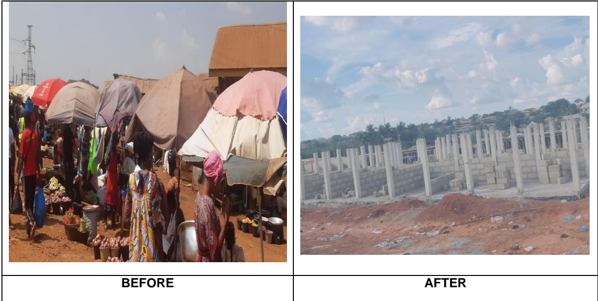
Construction of 108 Unit Market stalls, crèche, police post, fire hydrant and 1No Mechanized Borehole (Nana Bososma Market)
