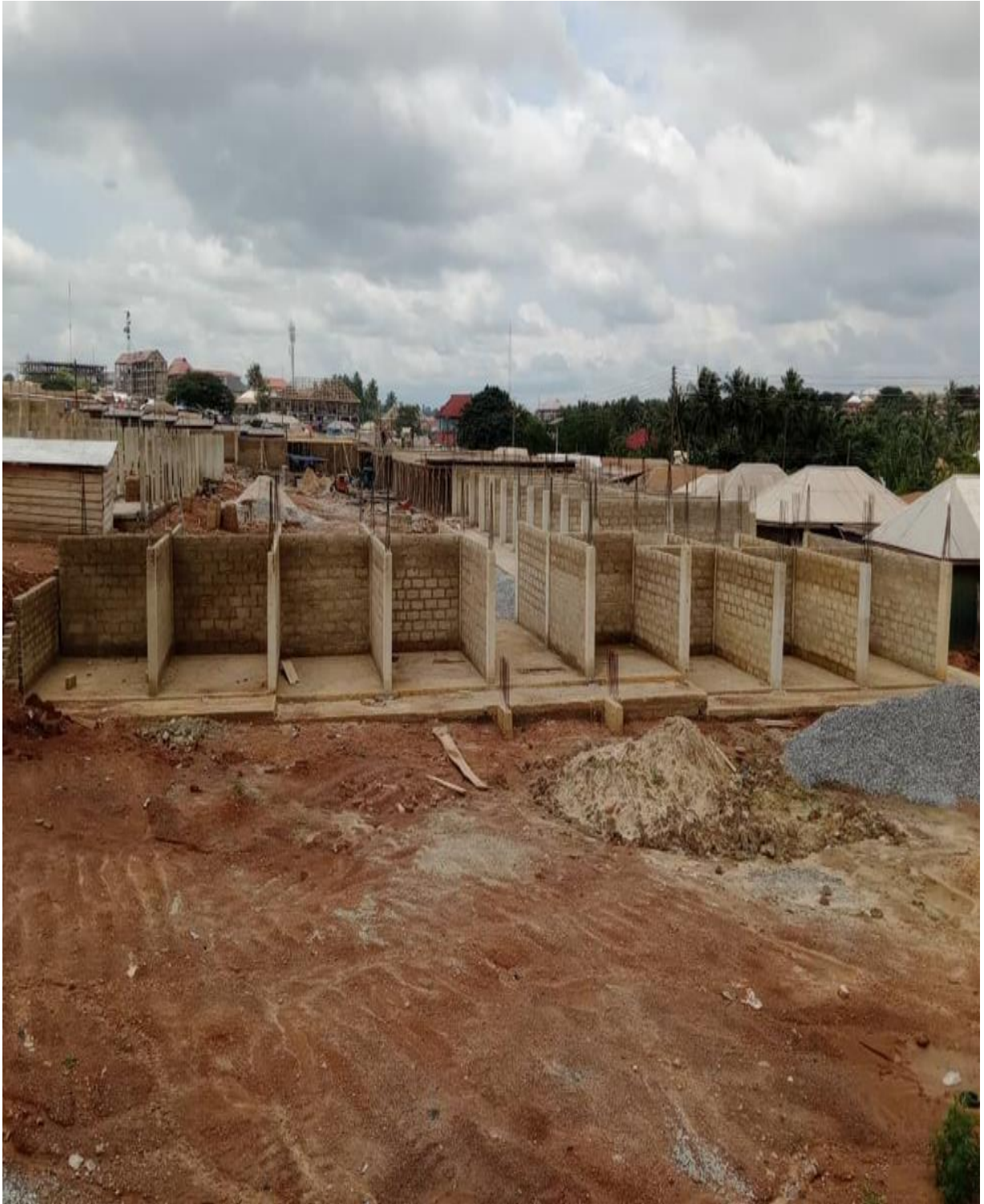
Construction of 96unit lockable store (phase 2) (Nana Bosoma Market)
