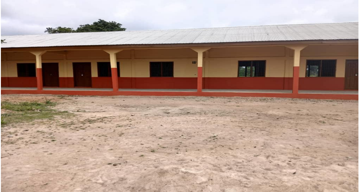
3 unit classroom Block constructed st Duadaso No.2 (IGF)
