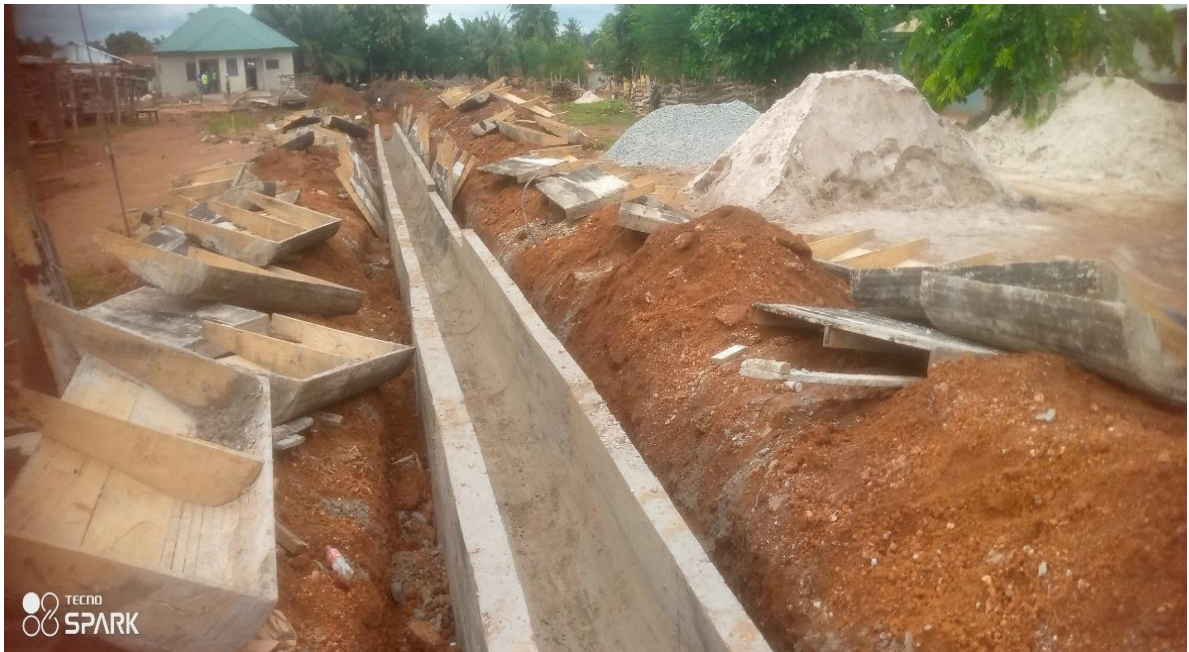
Picture 8: Upgrading 1.9Km Roads with Side Drains
