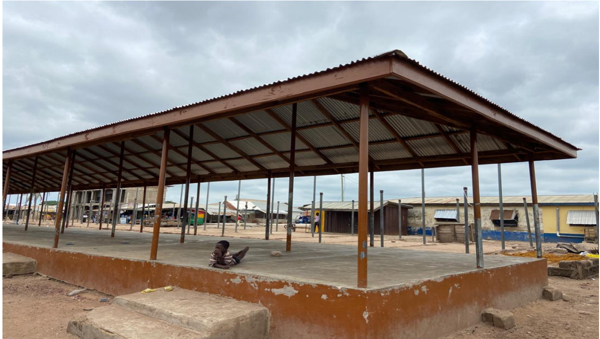
Completed the construction of a 50-unit market stalls at Yeji (DACF)
