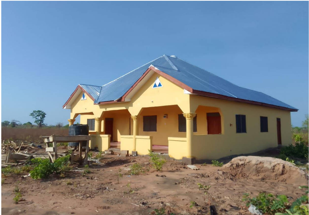
Completed the construction of CHPS Compound at Konkoma (DACF-RFG)
