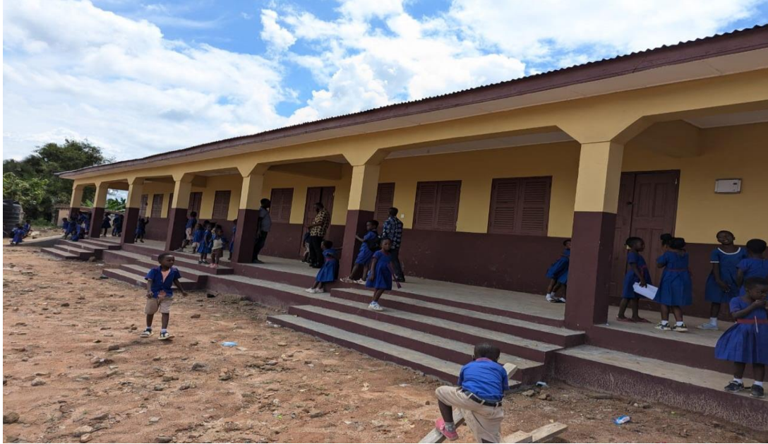
Constructed 1 No. 3 Unit Classroom with Office and Store at Ahamadyia Primary, Asokore
