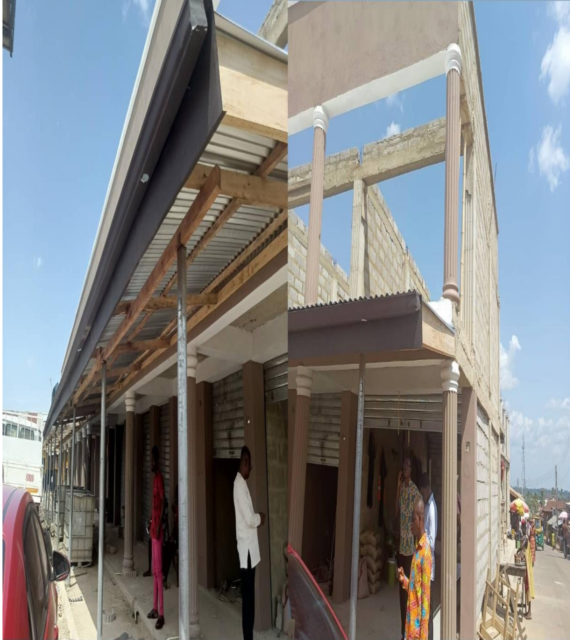
CONSTRUCTION OF 2 STOREY 120 MARKET STORES AT EFFIDUASE MARKET. FUNDING: PPA.
