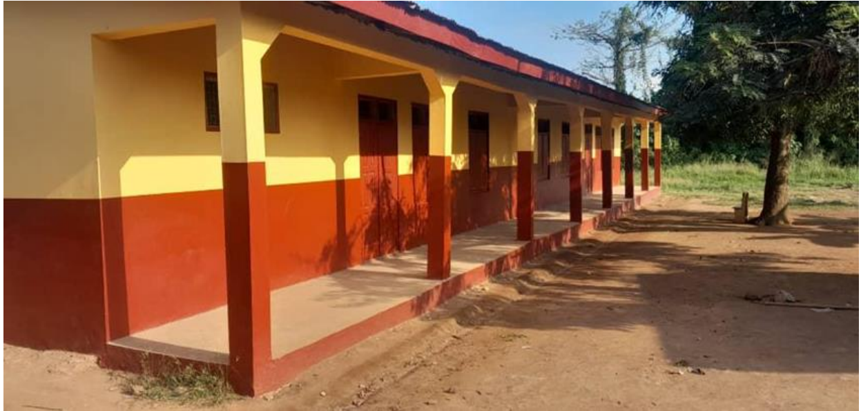
1 No. 3-Unit Classroom Block and 2No. Pavilions Completed at Apotosu (DACF
