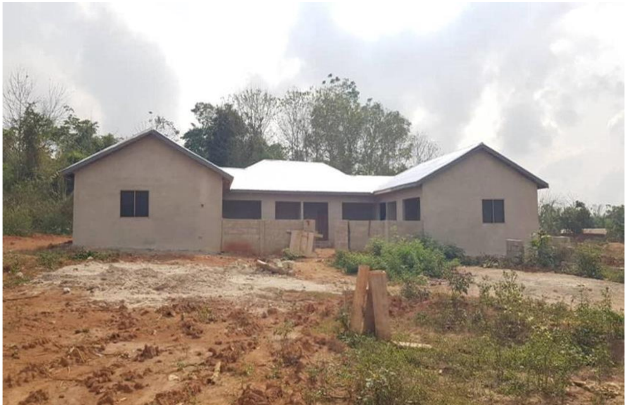
1No 6-unit Teachers Quarters constructed at Anhwerekrom (DPAT)
