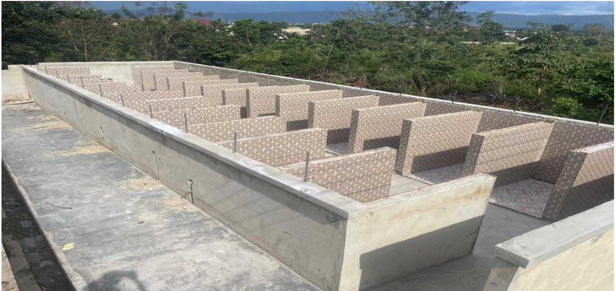
1NO. 24 UNIT BATHHOUSE AT CHRIST THE KING SHS 80% COMPLETED ,AKAPORISO
