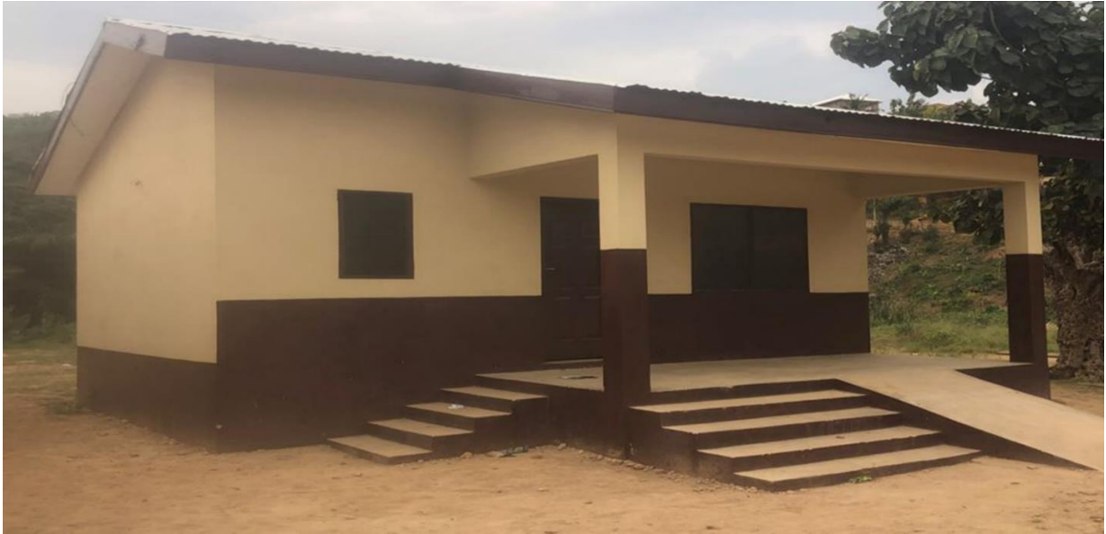
1NO. HEAD TEACHER'S OFFICE WITH WC STORE AND VERANDAH 100% COMPLETED AT AHANSONYEWODEA (IGF)
