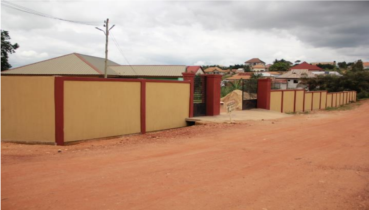
Fence wall, drainage and culvert constructed at Kunka health centre (IGF
