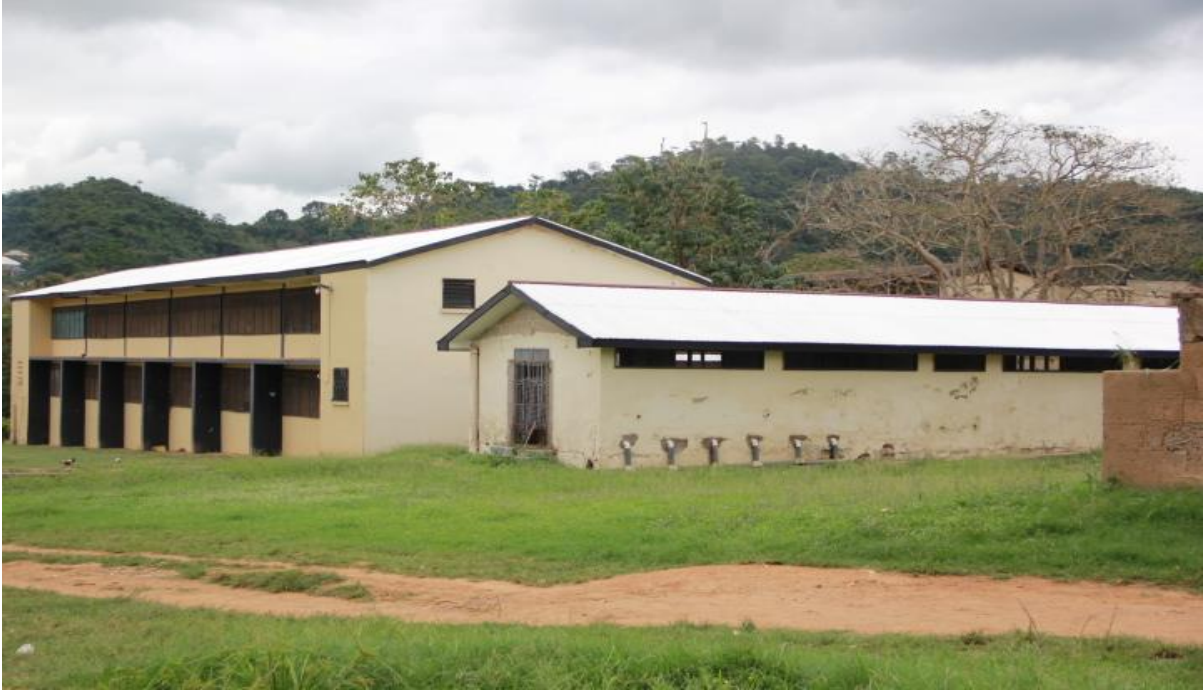
Dormitory, classroom block rehabilitated at Obuasi Senior high School (IGF)
