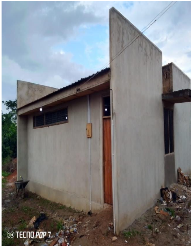
Seater WC toilet facility completed at Adaase (MPCF)
