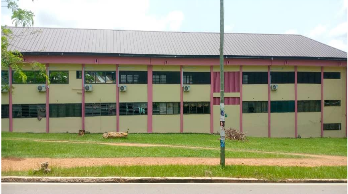
Main Assembly block renovated (Phase 1) (IGF)
