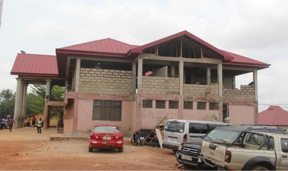
2-Storey Administration Block at Bantama Sub-metro at 70% completion - IGF
