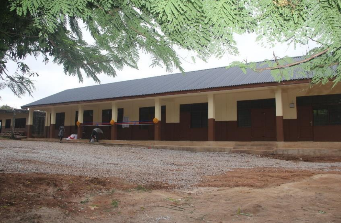
1No 3-unit Classroom Block at Abrepo M/A School Constructed - IGF
