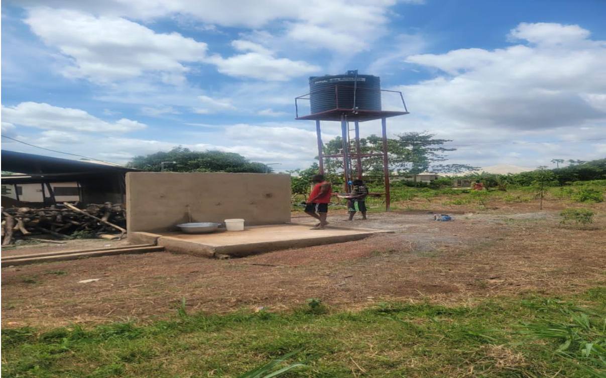
Mechanized borehole at Foase
