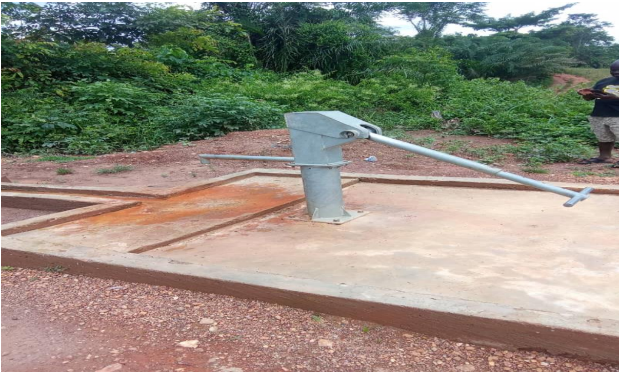
Borehole at Nkwanta
