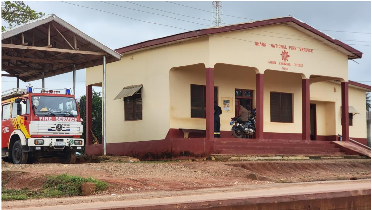
Old court renovated to fire service station
