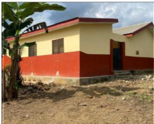
Mprakyire CHPS Nurses' Quarters (Source of Funding: DACF)
