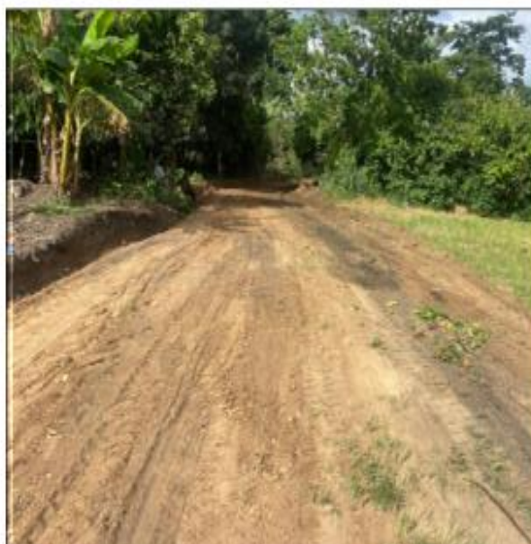
Abusa junction to Abusa 2km re-shaped road (Source of Funding: MPCF)
