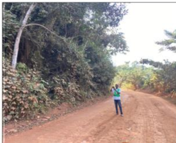
Kubi Junction to Kubi 5km re-shaped road (Source of Funding: MPCF)
