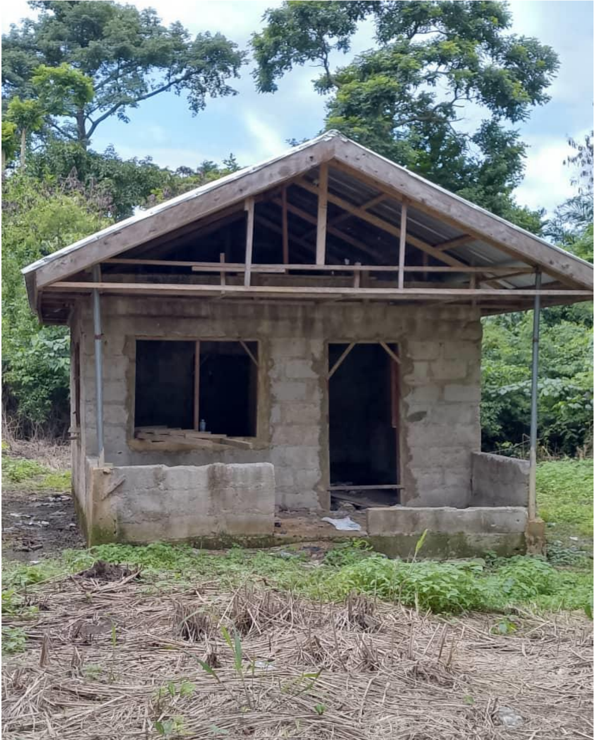
Constructed 1no. Police post at Kusi
