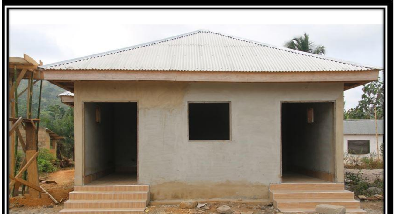
1 no.12-seater WC with mechanized borehole with overhead tank at Kusa
