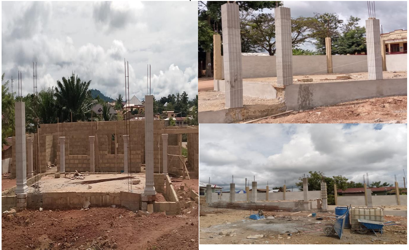
Constructed of 1no. Durbar Ground at Dompase
