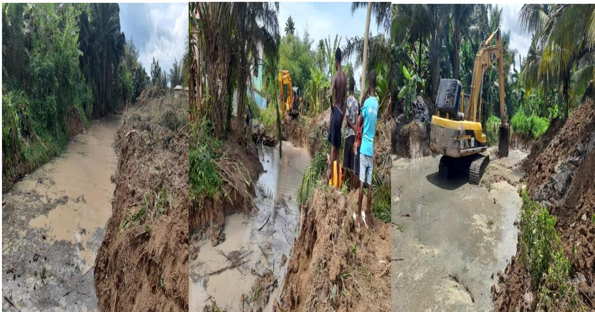
Dredged Evaley & Ayile Storm Drains 2.1km and Dredged Effia Storm Drain to a distance of 1.2km
