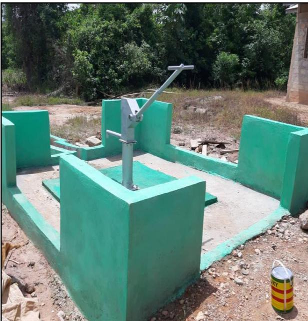
Constructed 3 No. Boreholes fitted with Hand Pumps and Dwarf Walling at Ethiopia Forest
