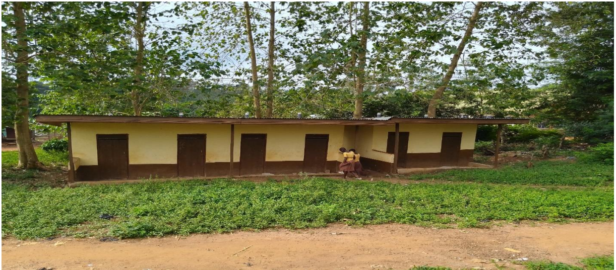
Constructed 1No. 6 Se6-Seater VIPIlet at Juaboso Cluster of Schools
