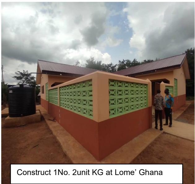
Construct 1No. 2unit KG at Lome' Ghana
