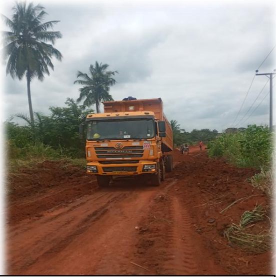
Reshaping of 0.85km roads
