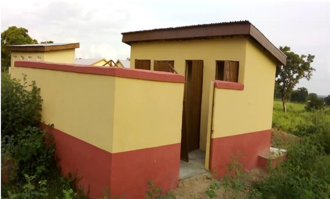
Constructed 2-unit KVIP toilet and urinal at Holomoni
