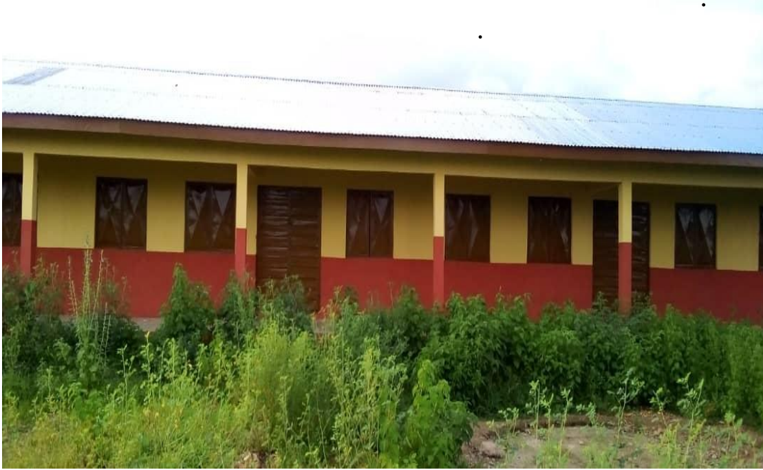
Constructed 1No. 3Unit Classroom Block, Staff Room, store
