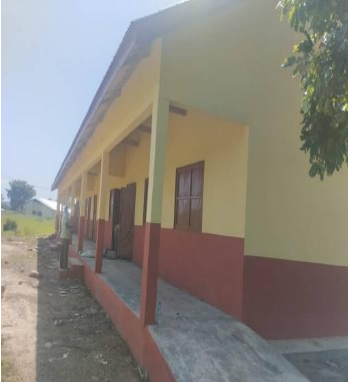
3 Unit Classroom Block at Kaa Ongoing
