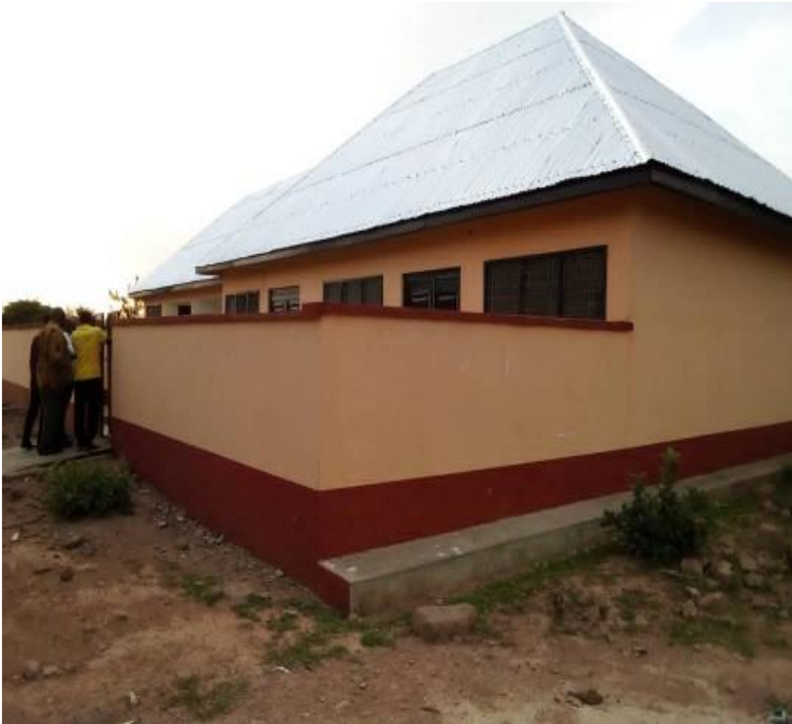
CHPS Compound at Liplime– Completed and Handed Over
