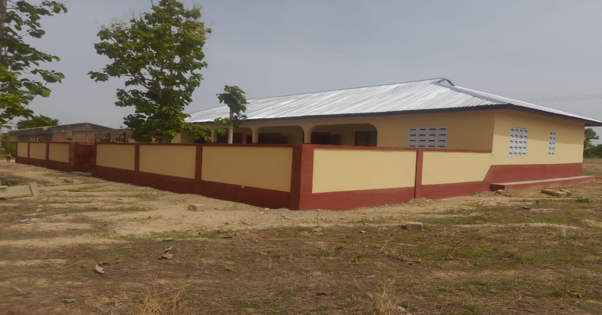
Figure 4: Constructed and Furnished 1No. KG Block at Domange
