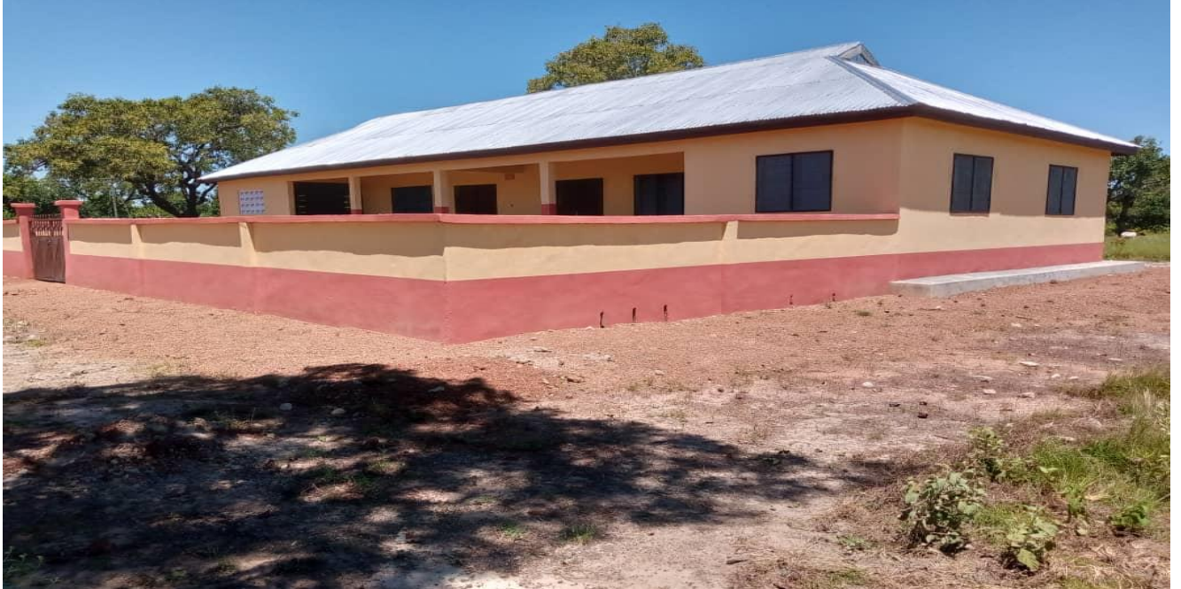
Figure 2: Constructed and Furnished 1no. KG Block at Bekyiteng
