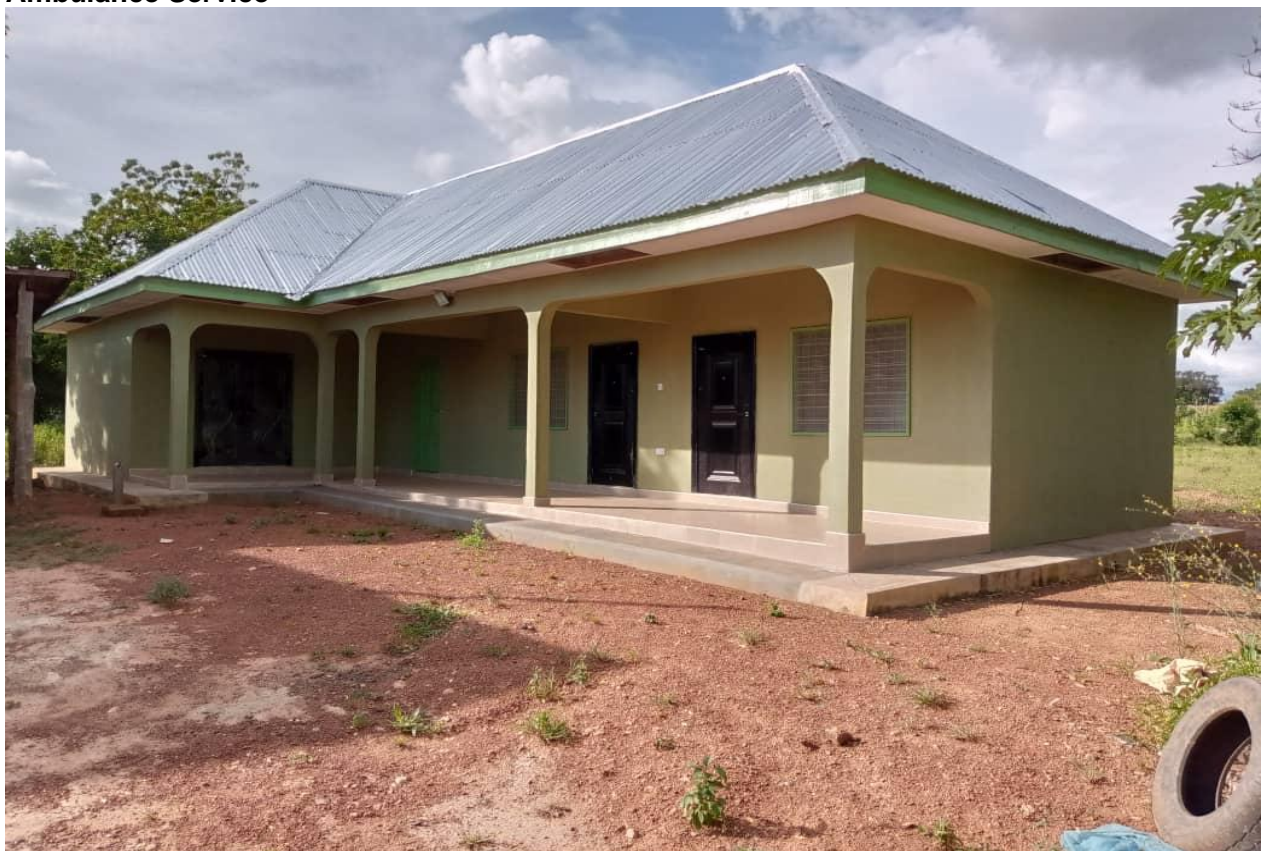
Figure 1: Constructed and Furnished 1No. Office Complex and ancillary facilities for Ambulance Service
