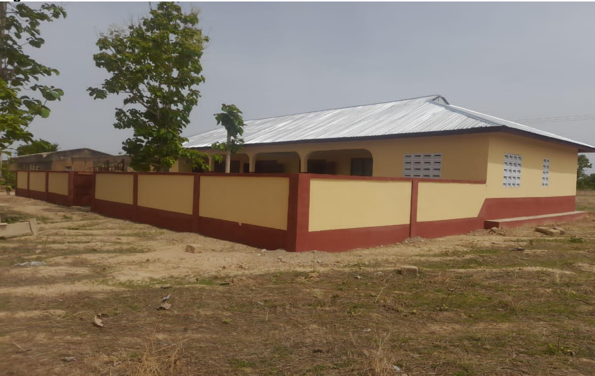
Figure 5: Constructed and Furnished 1No. KG Block at Bu
