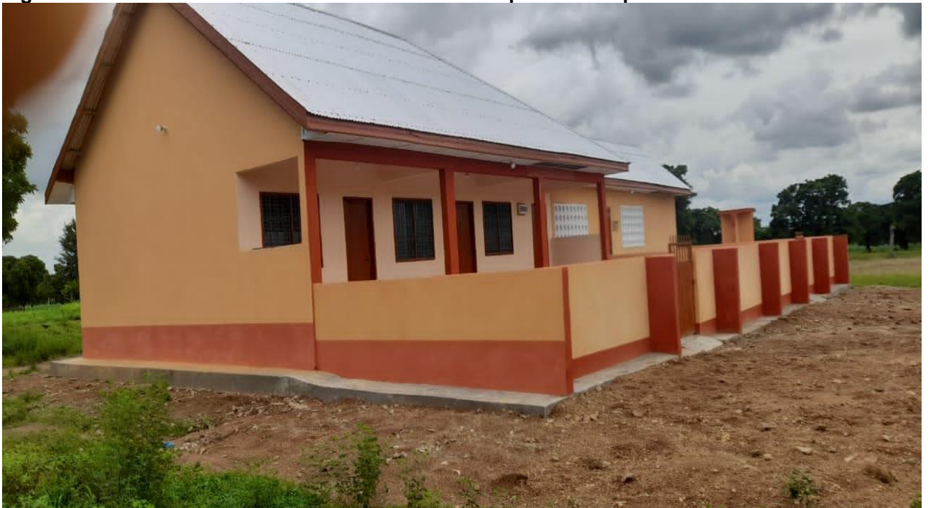
Figure 3: Constructed and Furnished 1no. CHPS Compound at Vapuo
