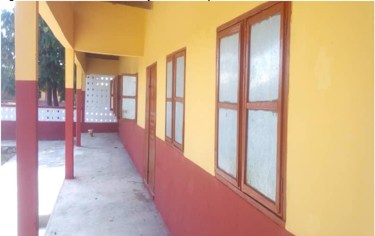
Figure 7: Rehabilitated 1No. Primary School at Bapula
