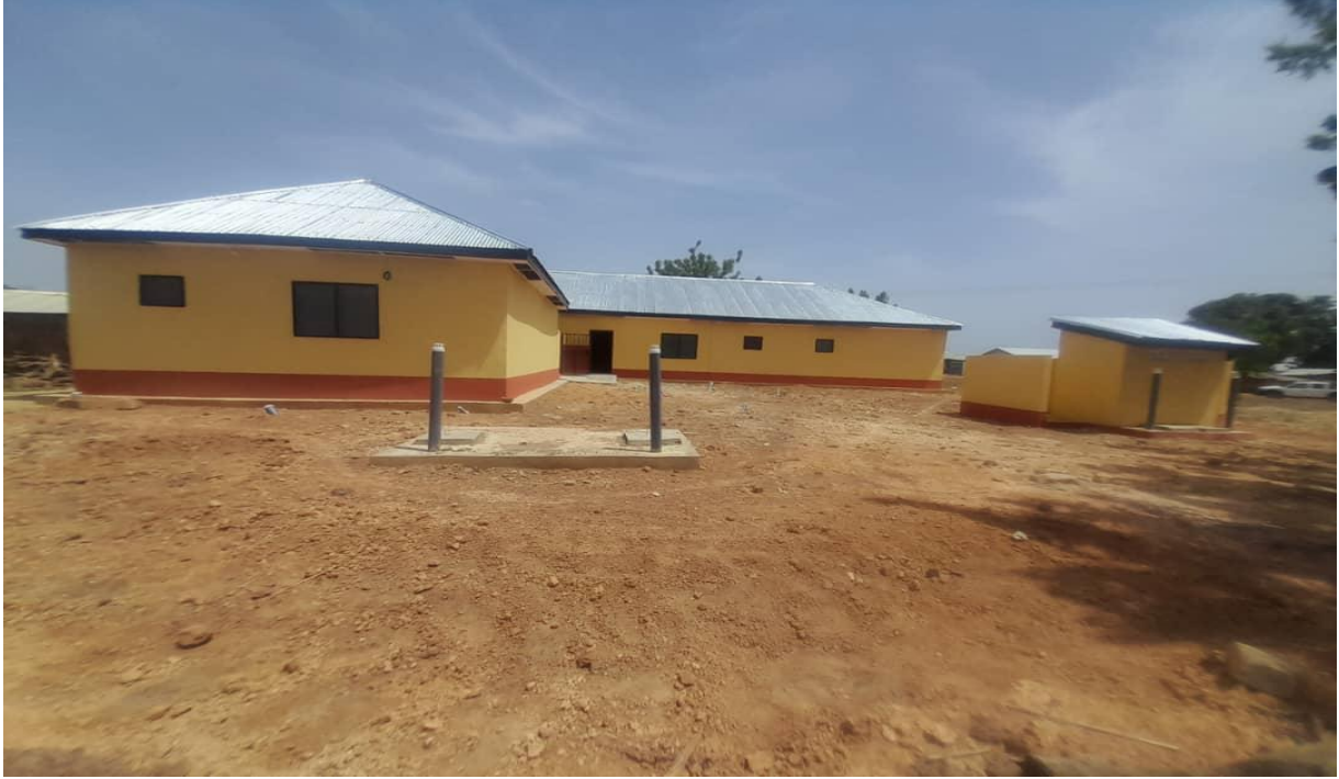
Figure 6: Constructed and Furnished 1No. CHPS Compound at Tantuo
