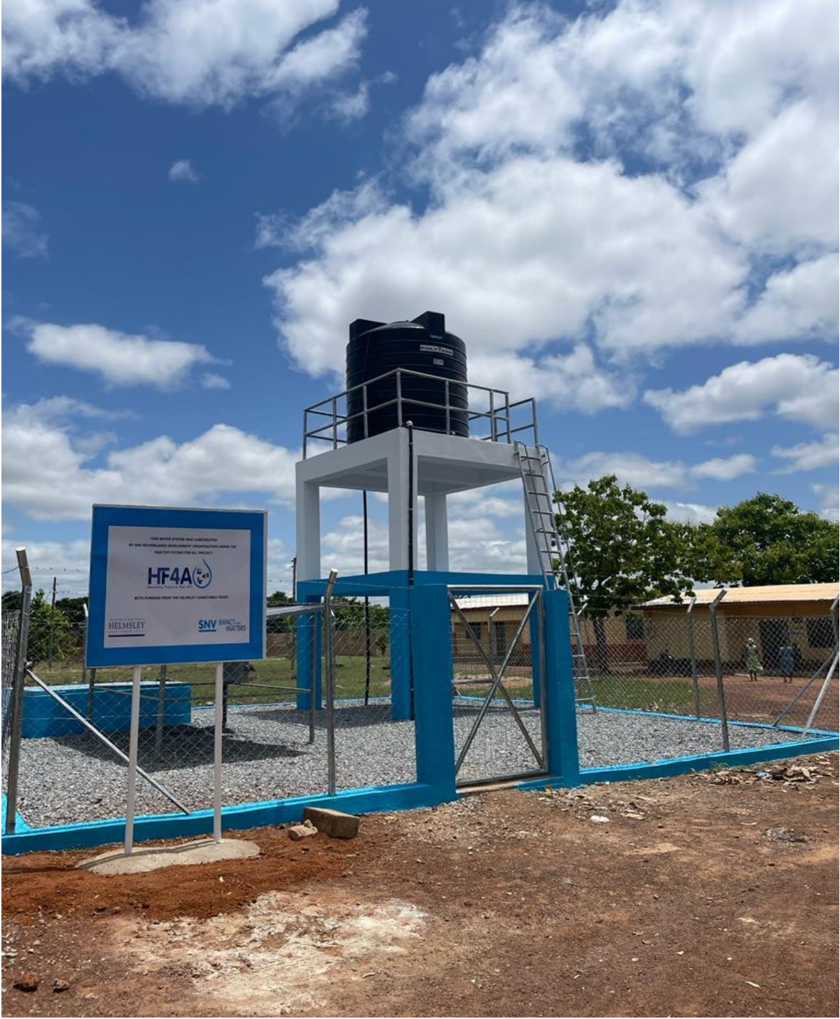
Figure 8: Solar Powered Limited Water System piped into Health Facility and community at Piiri, supported by SNV
