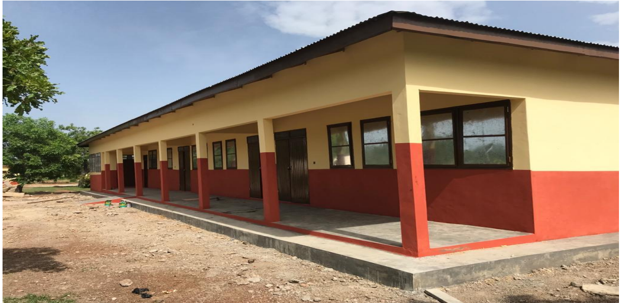
CONSTRUCTED AND FURNISHED 1NO. 3-UNIT CLASSROOM BLOCK AT FIAN
