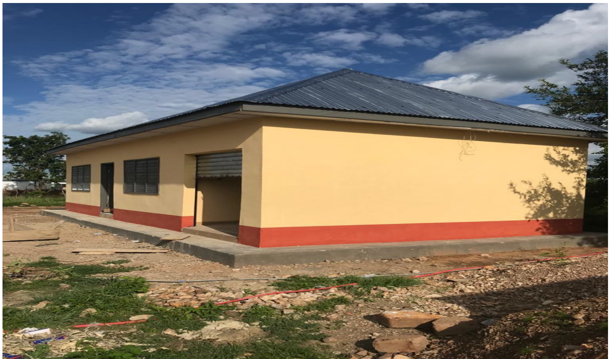
CONSTRUCTED AND EXPANDED 1NO. FIRE SERVICE ACCOMODATION WITH A BAY AT ISSA
