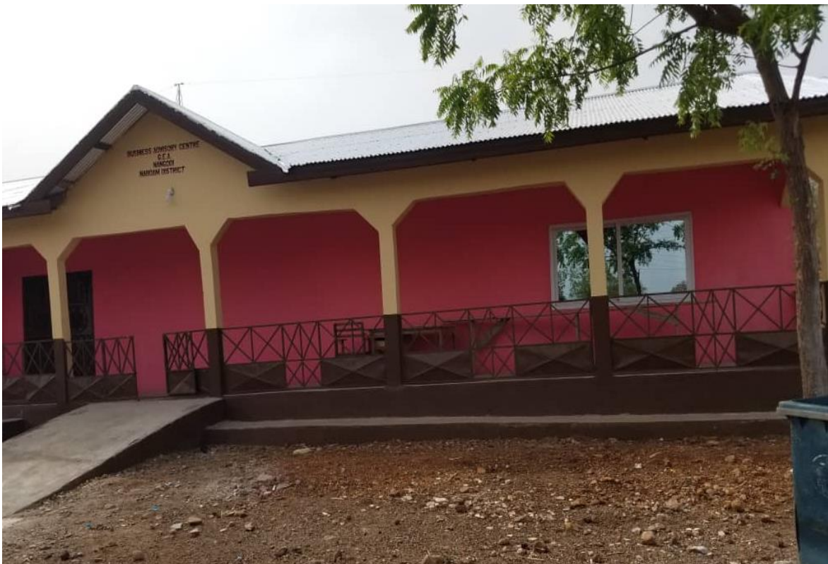
Completed the construction of the Business Adversary Centre District Office
