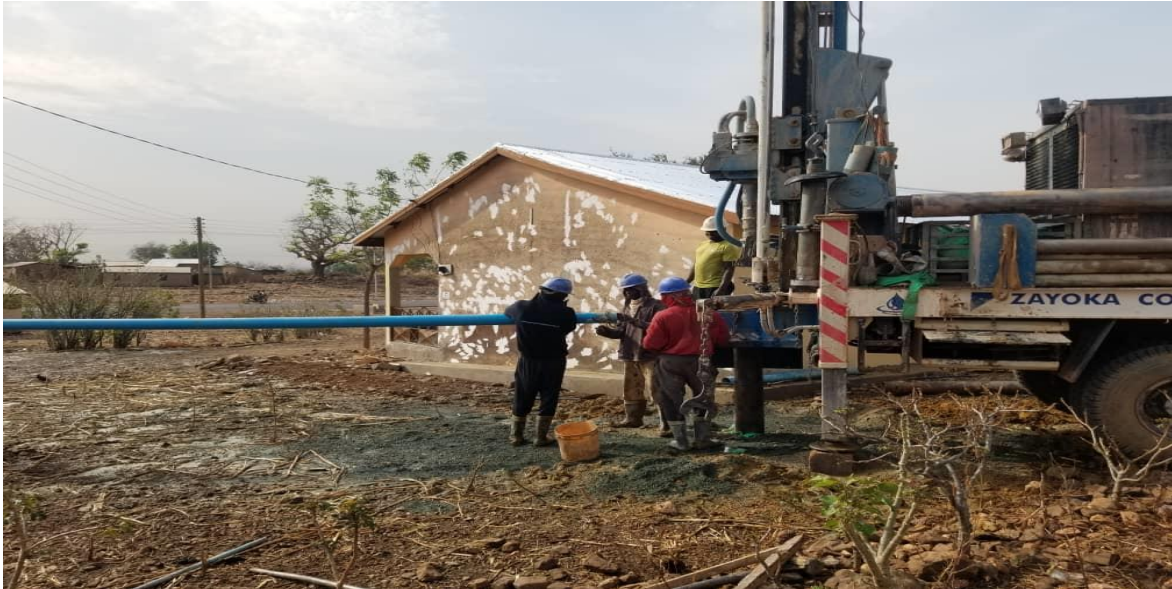
Drilled 1No borehole at the Business Advisory Centre District Office
