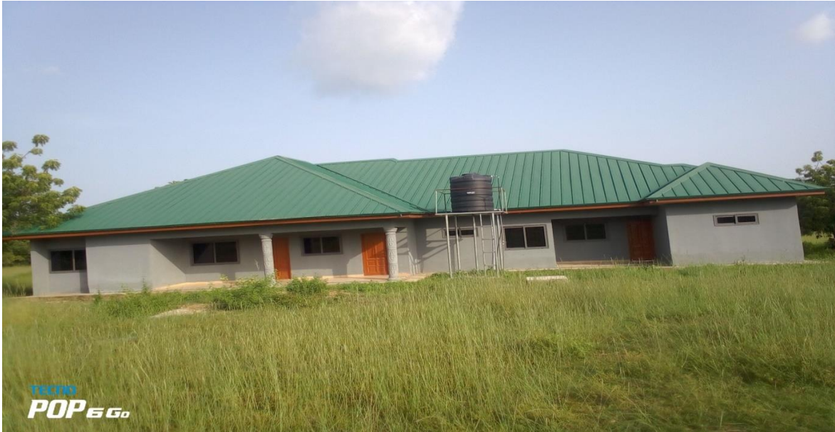
DCE Bungalow constructed-DACF-RFG
