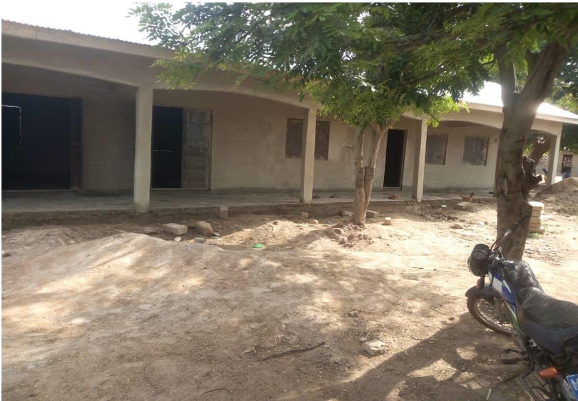
Construction of 1No 3-Unit classroom block at Nyogbare-DACF-RFG
