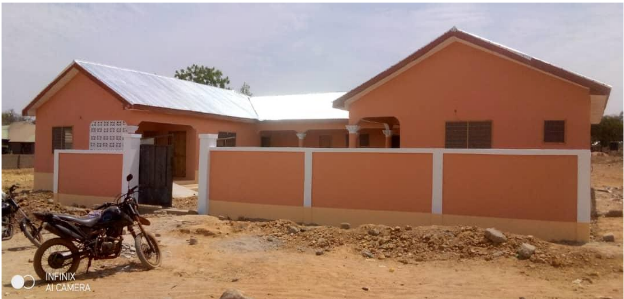
Constructed ICT and Library block with ancillary facilities at Chuchuliga (DACF-RFG)
