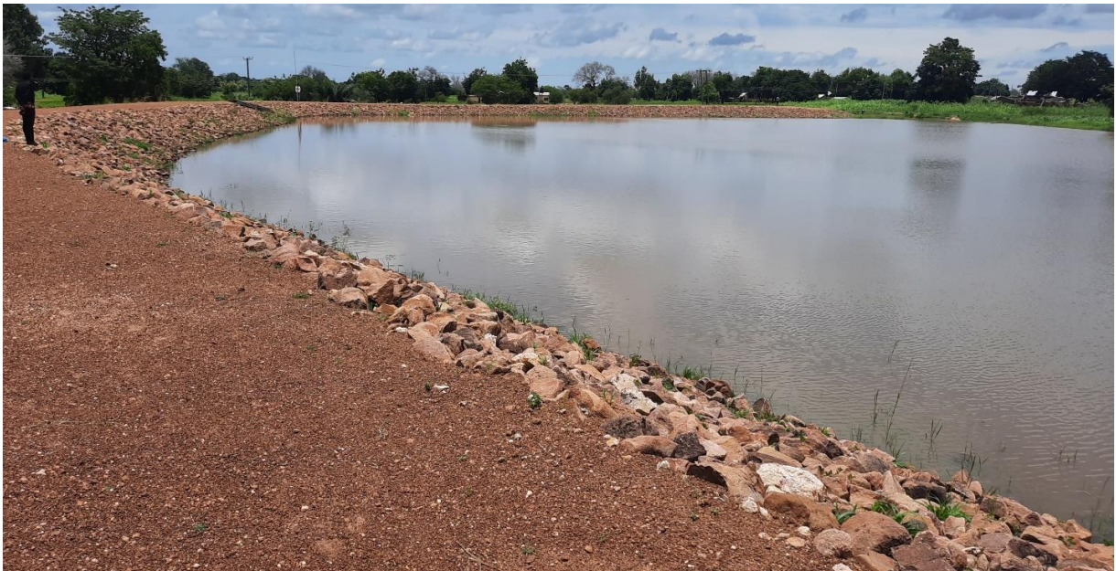
Rehabilitated 1no. Small Earth Dam at Kalijisa (GPSNP)
