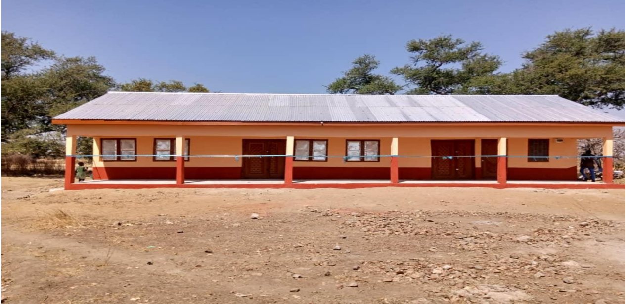
Completed KG block at Kpandema (MPCF)
