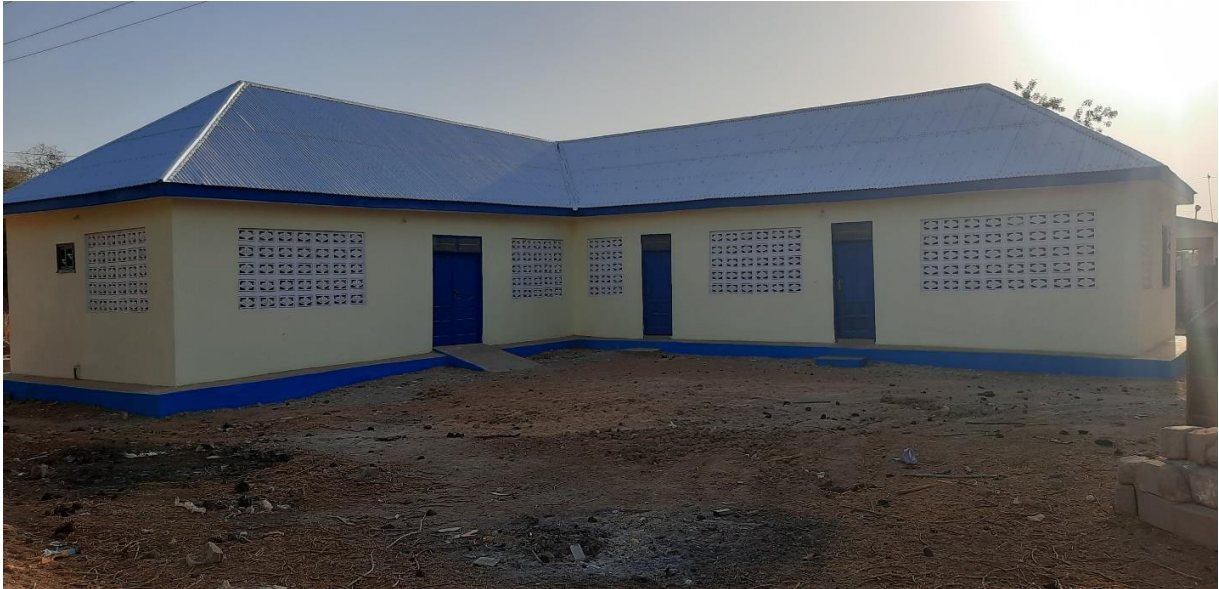
Constructed office block with ancillary facilities for the Municipal Health Insurance Scheme at Sandema (DACF-RFG)
