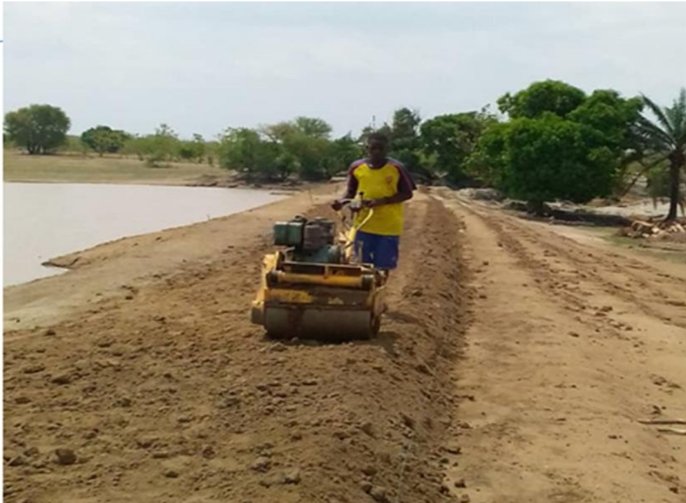
Construction of Arizeem Dam
