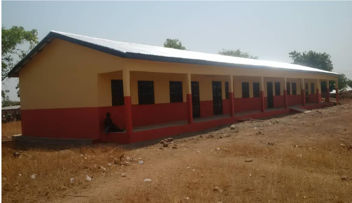
Fig. 1.1 Constructed 1No. 3-unit classroom block at Nabengu
