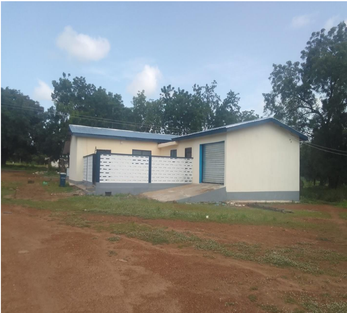
REHABILITATED AGRIC. DIRECTOR BUNGALOW
