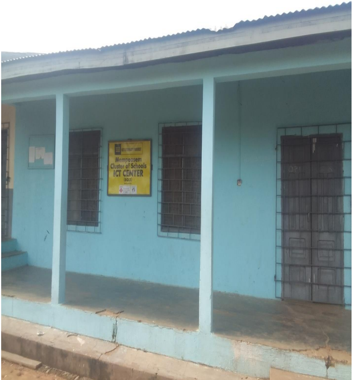
REHABILITATED CLUSTER OF SCHOOL ICT CENTRE AT MEPEASEM
