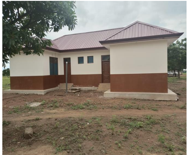
CHPS compounds at Kadia
