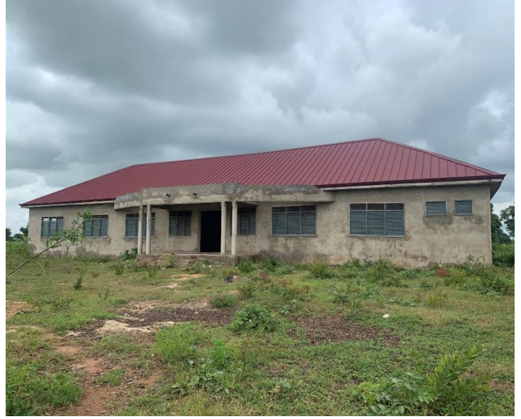
Construction of 1 No. Agric Directorate with Vet Lab at Nanton (Plastered)
