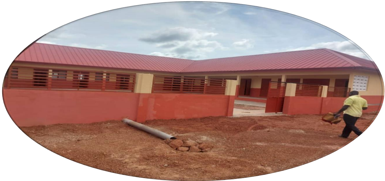
Constructed 1 No. Girls Model School at Nanton (Completed)
