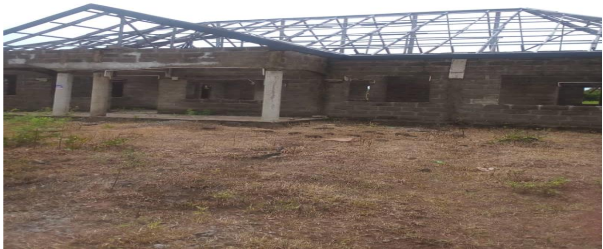
Construction of 1No. CHPS Compound at Kpunduli (Roofing level)
