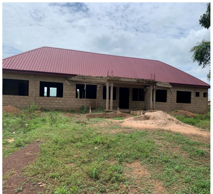
Construction of 1 No. GES Directorate at Nanton (Roofed)
