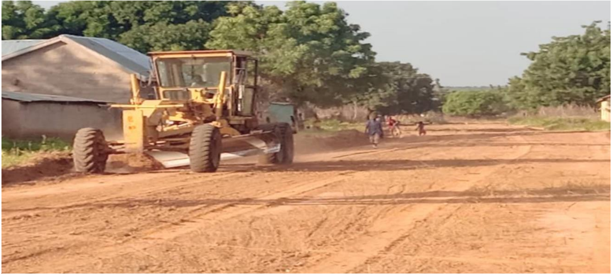
ENGINEERED UPTO 10KM ROAD IN THE KUMBUNGU TOWNSHIP
