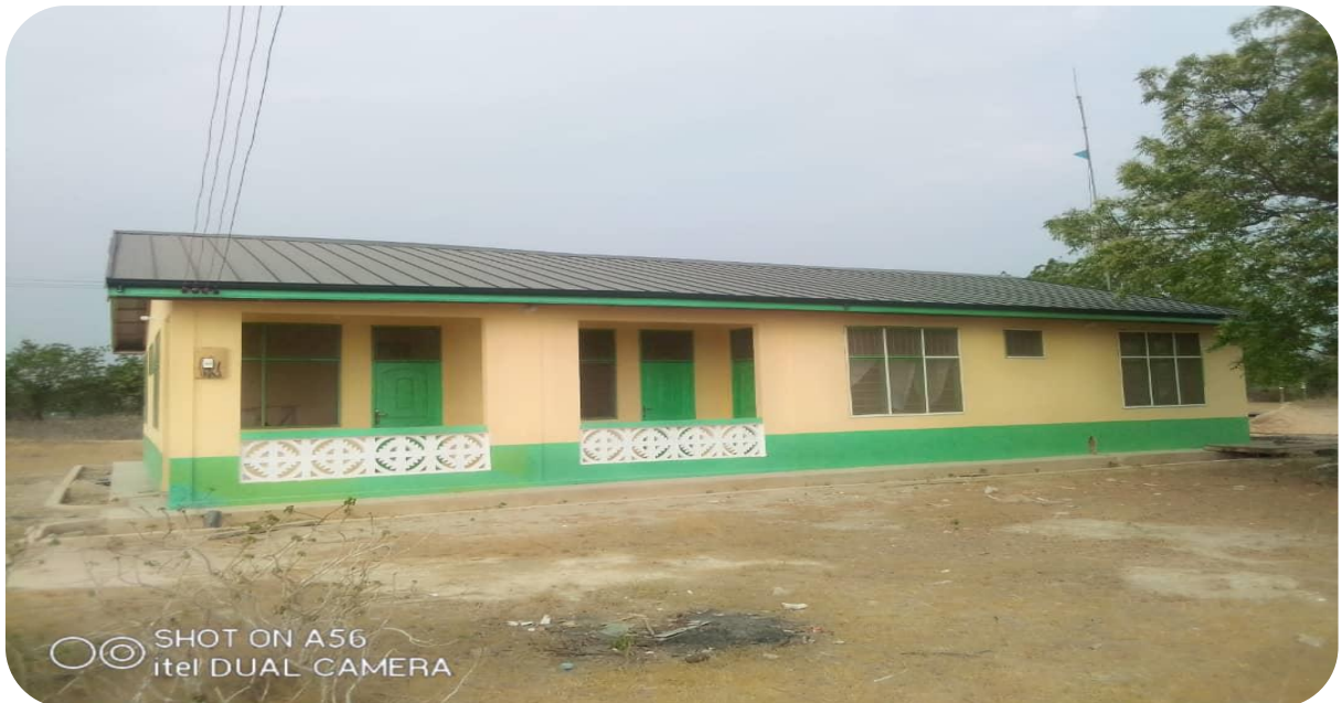
Agortor CHPS Compound
