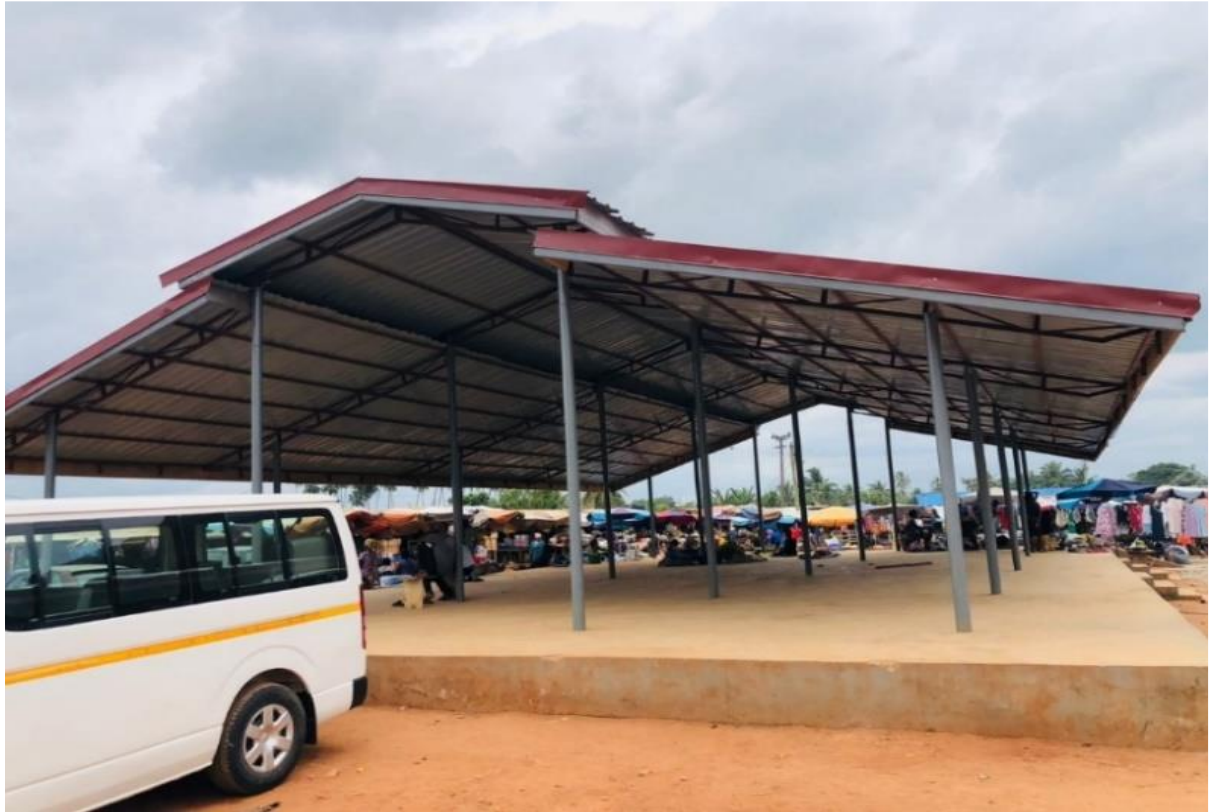
Completed 2No. 36 open shed at Dodowa Market
