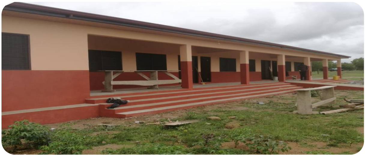
3-Unit classroom Block at Huapa
