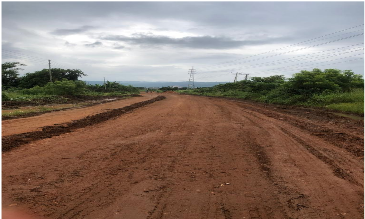
Reshaped and Graveled Ashiaman Junction-SOTA Road.
