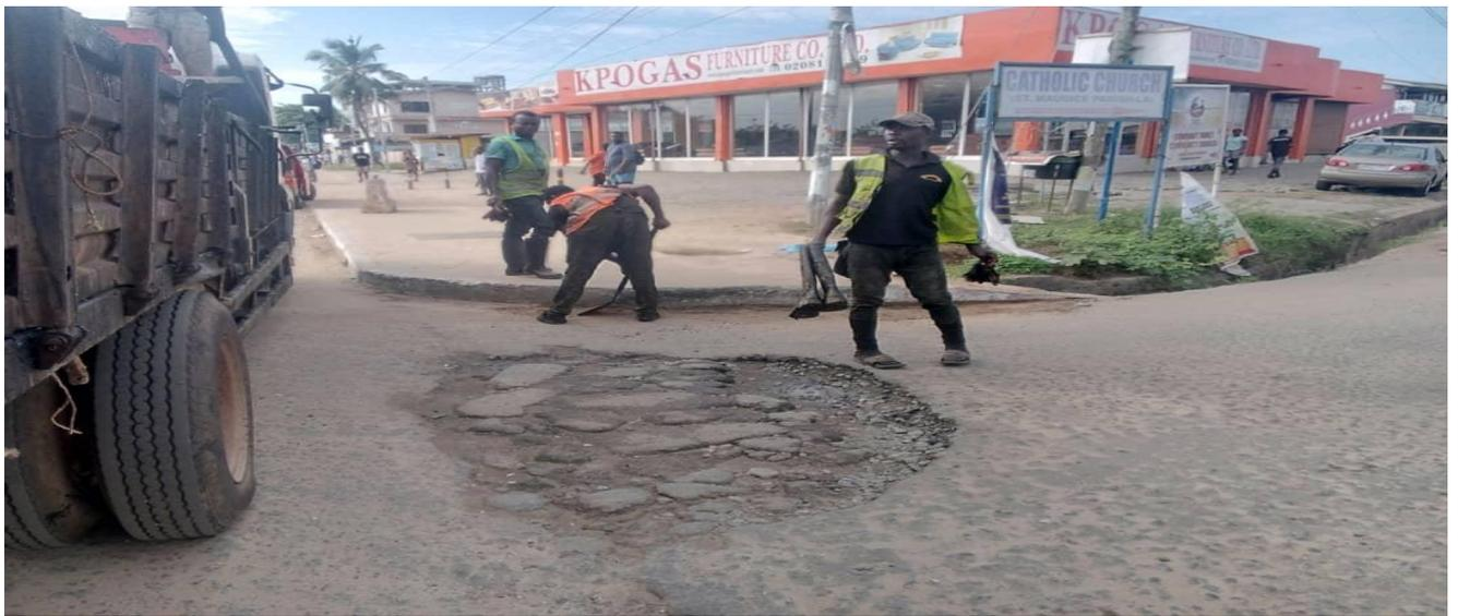
**FIGURE 7 POT HOLE PATCHING WITHIN THE MUNICIPALITY**
